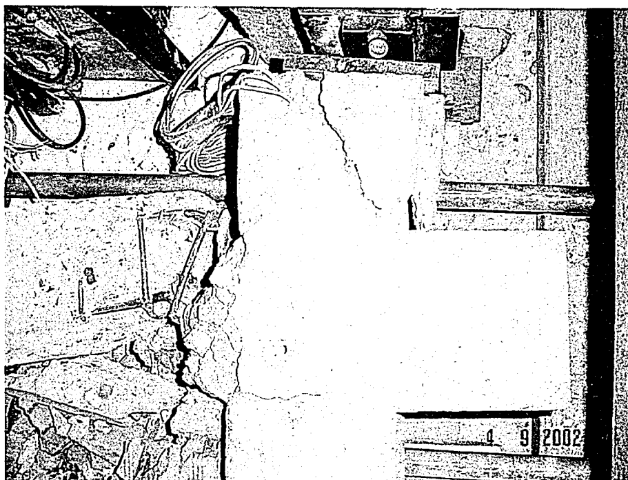
Figure 4.10. Crushed column end zone of 01NC-IN
