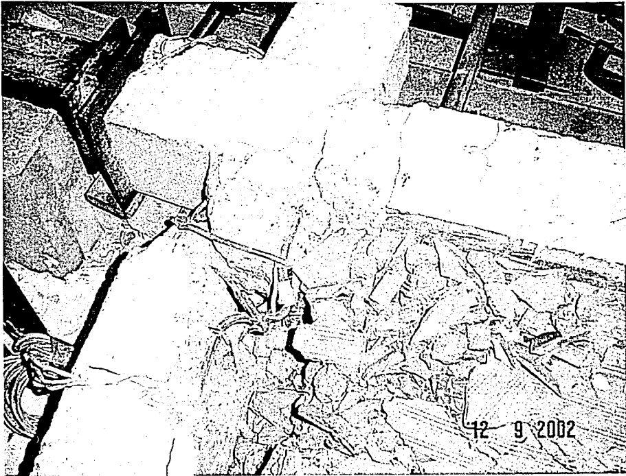
Figure 4.13. Crushed column end zone and buckled reinforcement
