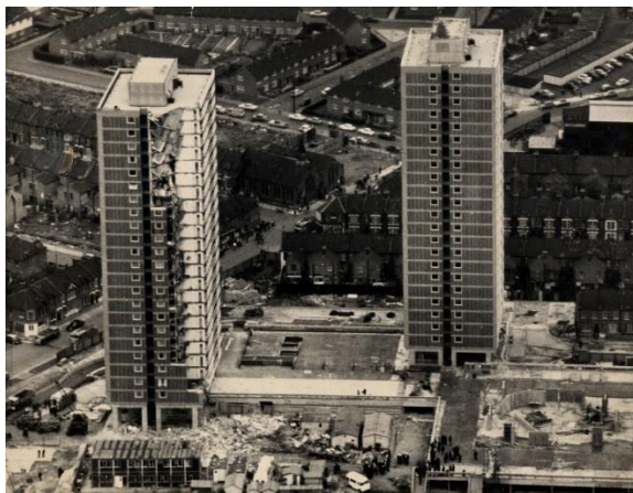
Figure 2.1. Ronan Point accident.
