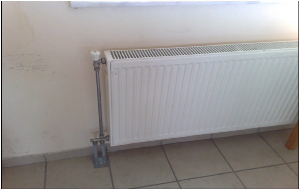
Figure 2.5. Radiator Valves.
