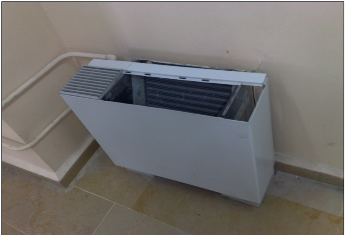
Figure 2.6. Fan Coils.
