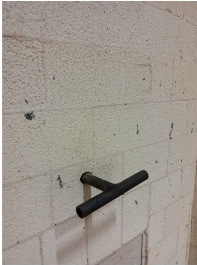
Figure 3.6. Pressure sensor from inside the furnace.
