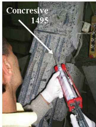
Epoxy injection of large cracks
