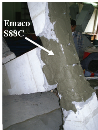
Replacement of loose concrete voids
