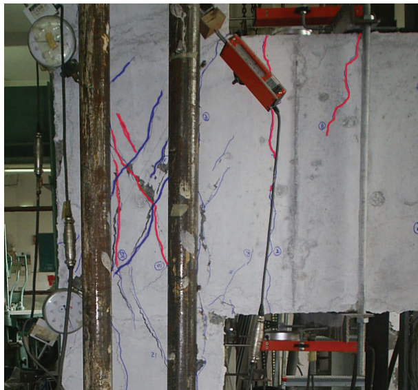
Figure 5.22. Shear failure at the joint core
