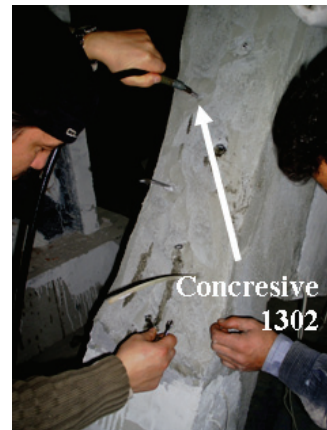
High-pressure epoxy injection
