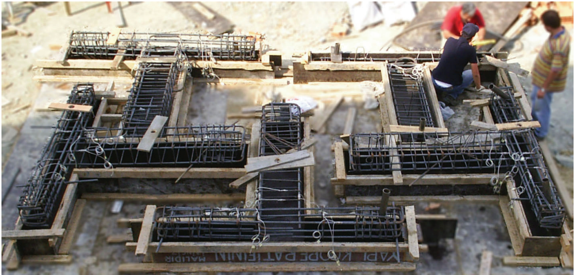
Figure 3.2. Construction of the specimens
