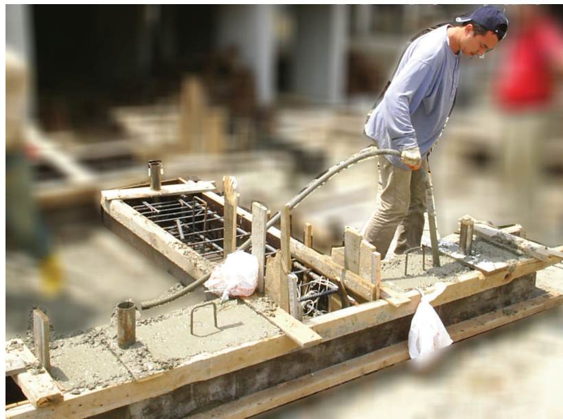
Figure 3.3. Use of immerse vibrator
