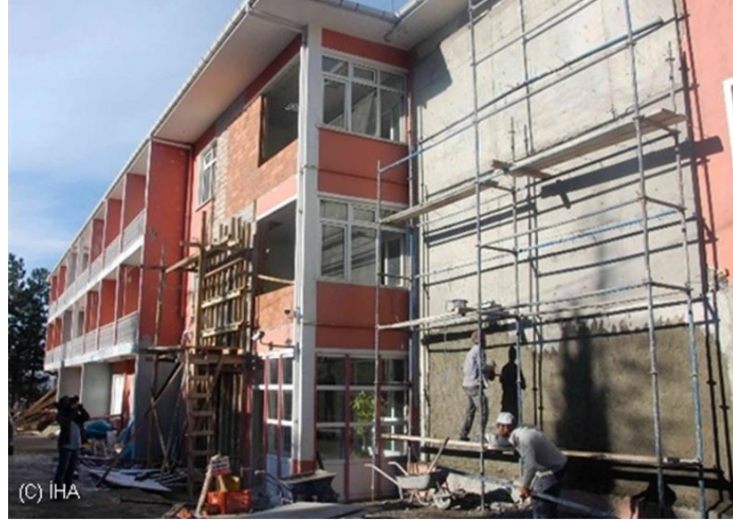
Figure 6.1. Retrofitting of a hospital.
