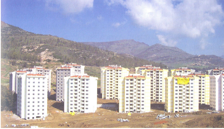
Fig. 14 Örnekköy Gecekondu Transformation Area after transformation
