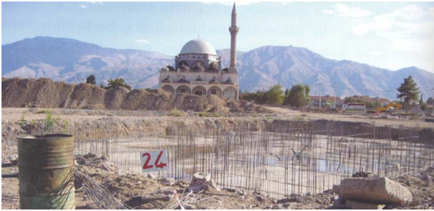
Fig. 10 Erzincan Çarşı Gecekondu Transformation Area during transformation
