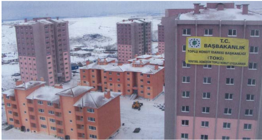
Fig. 6 Airport Highway after transformation
