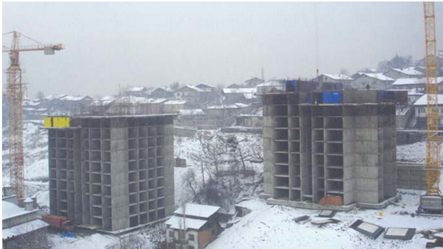
Fig. 13 Karabük Cevizli Gecekondu Transformation Area during transformation
