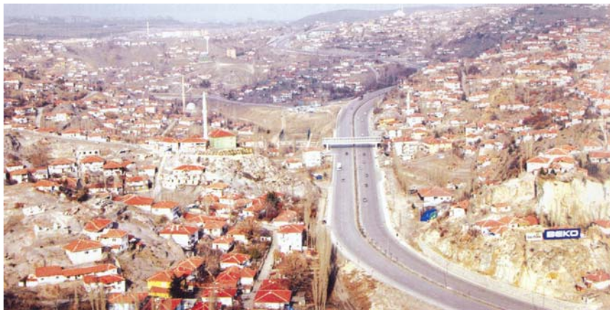
Fig.4 Airport Highway before transformation 243
