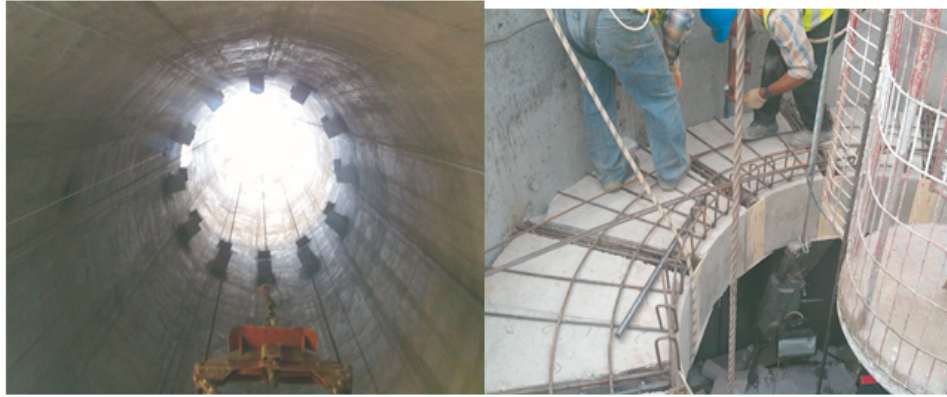
Figure 2.4. Precast Slabs and Corbels.
