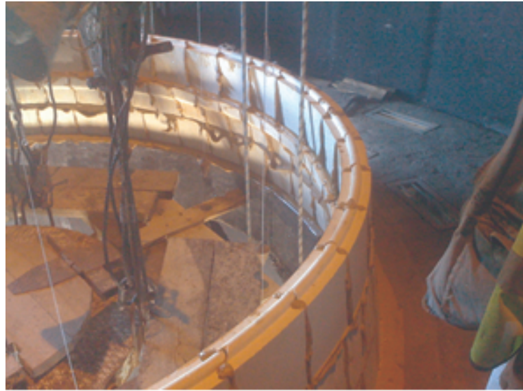
Figure 1.4. Brick Liner Construction on Precast Slabs (ENDEM Co.).
