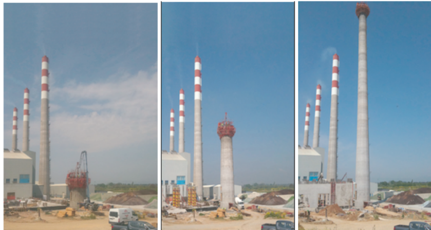
Figure 1.8. Construction Phase of the Chimney (ENDEM Co.).
