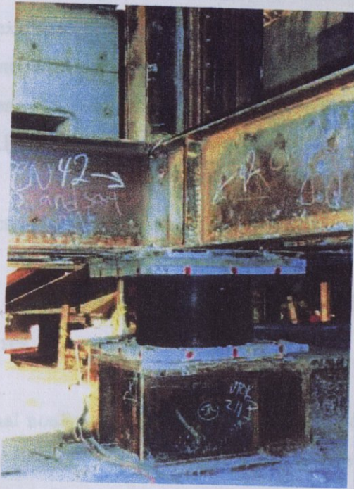
Figure 3.10. An application of a lead-plug isolator
