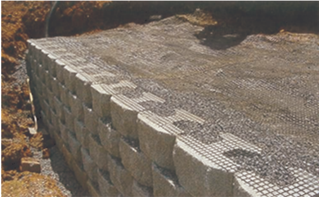
Figure 2.5. Modular block facing with geogrid reinforcement.
