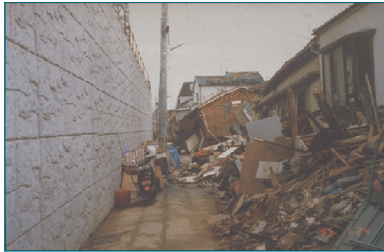
Figure 2.17. Tanata Wall and the around structures after Kobe Earthquake.
