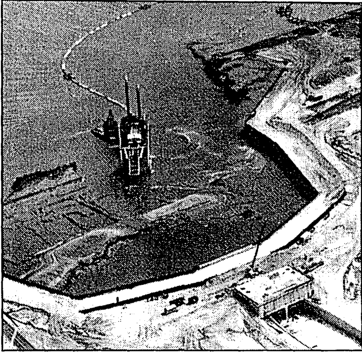
FIGURE 20.4. DREDGING NEAR THE RIVER BANKS (Courtesy of J. Krokeborg, 1990)
