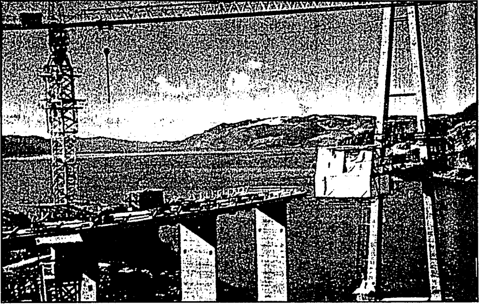
FIGURE 10.6. ERECTION OF THE GIRDER ( Courtesy of S. Vegvesen, 1994 )
