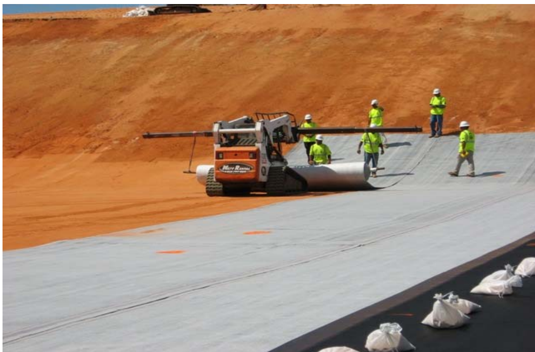
Figure 2.2. Deployment of GCL with a group of laborers (Greg Richardson et al., 2002)
