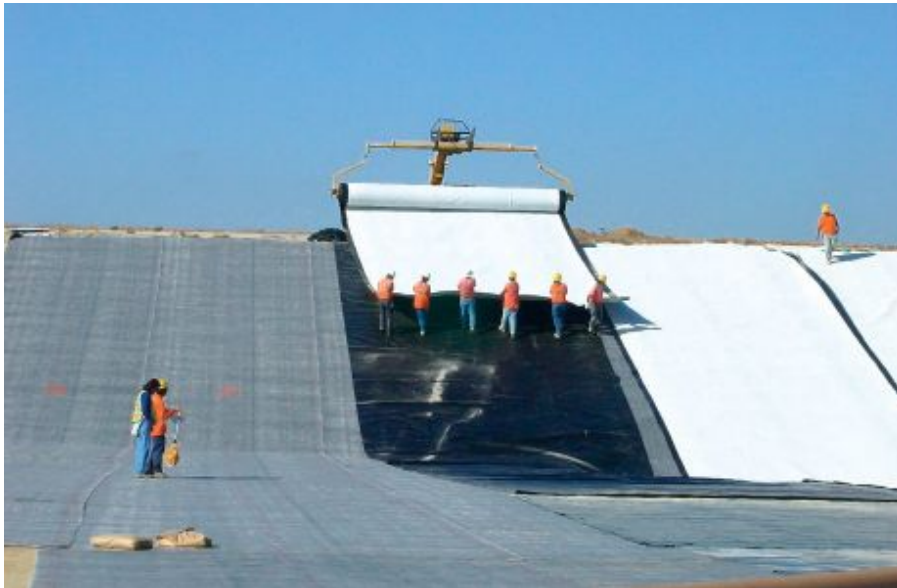
Figure 2.4. Unrolling of GCL on a slope (Greg Richardson et al., 2002)
