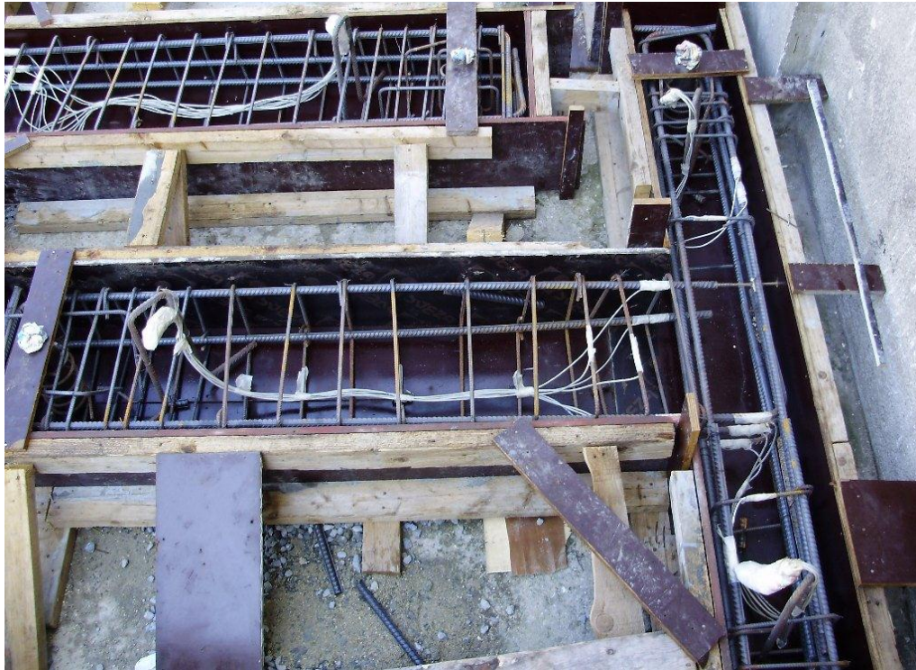
Figure 2.6. A picture of US3-FRP1 and US3-FRP2 from the construction site
