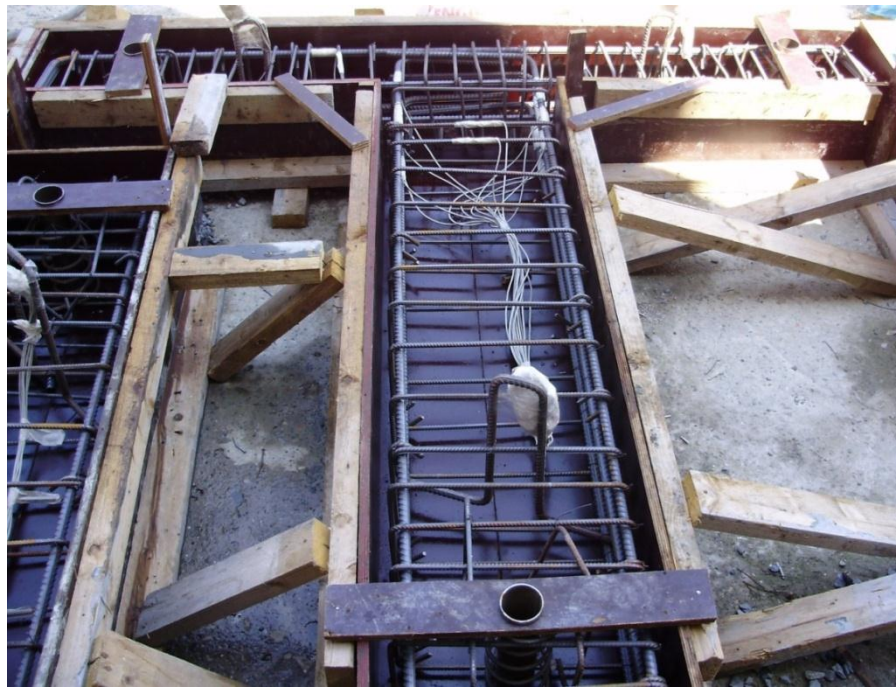
Figure 2.4. A picture of US3-ACI from the construction site
