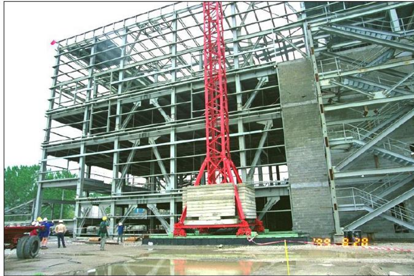
Figure 4.2. Example of EBF application (SEAOC 2000)
