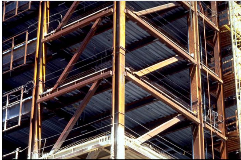
Figure 4.4. Example of EBF application (SEAOC 2000)
