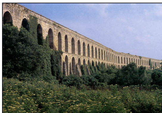
Figure 2.9. Uzunkemer Aqueduct, Turkey [31]
