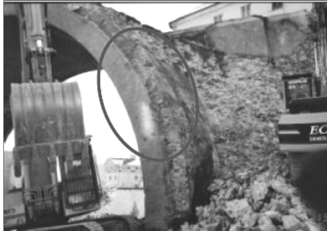
Figure 4.3. Changing in the thickness of voussoir [44]
