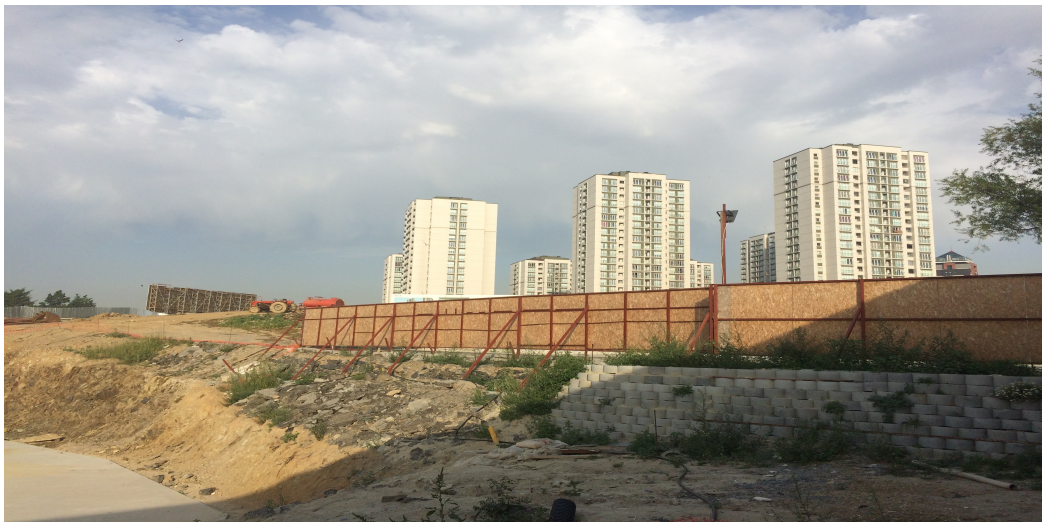
Figure 5.5. The construction site in Karayolları neighborhood.
