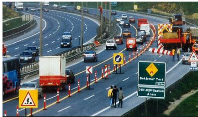
Figure 2.3. An Example of Vertical Marking
