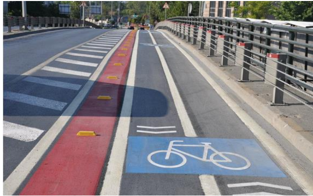
Figure 2.2. An Example of Horizontal Marking
