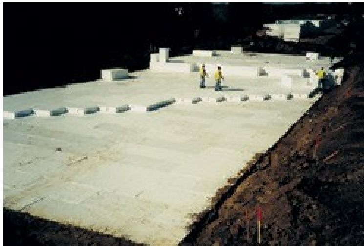
Figure 2.1. Construction of geofilm road embankment
