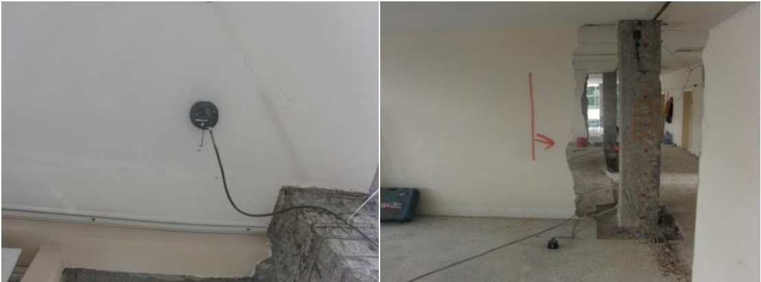
Figure 4.3. Accelerometers Affixed on the Slabs Near Columns.
