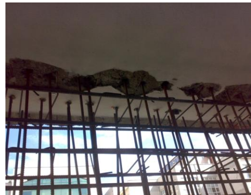
Figures 3.11. Vertical Anchor Bars Epoxied into Holes Drilled in Beams.
