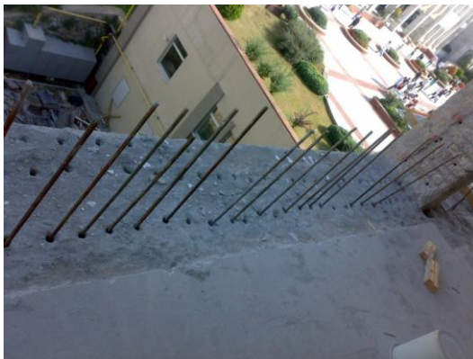
Figures 3.11. Vertical Anchor Bars Epoxied into Holes Drilled in Beams.
