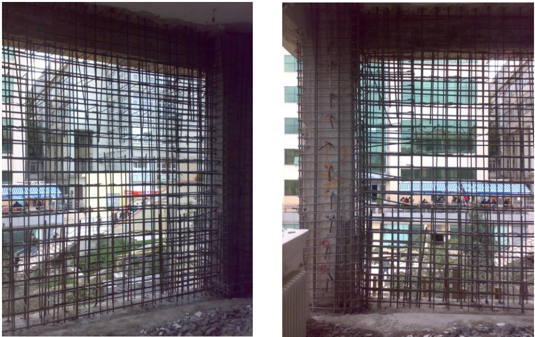
Figure 3.12. Reinforcement Details for Additional Structural Walls.
