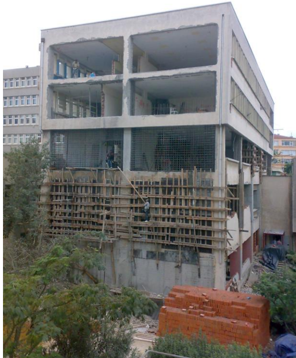
Figure 3.4. View of the Building during Strengthening, from East.
