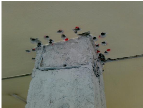
Figure 3.8. Holes Drilled in Slab for Continuation of Longitudinal Reinforcement.
