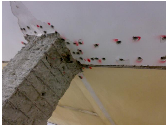
Figure 3.10. Preparation of the Wall Boundary Column.
