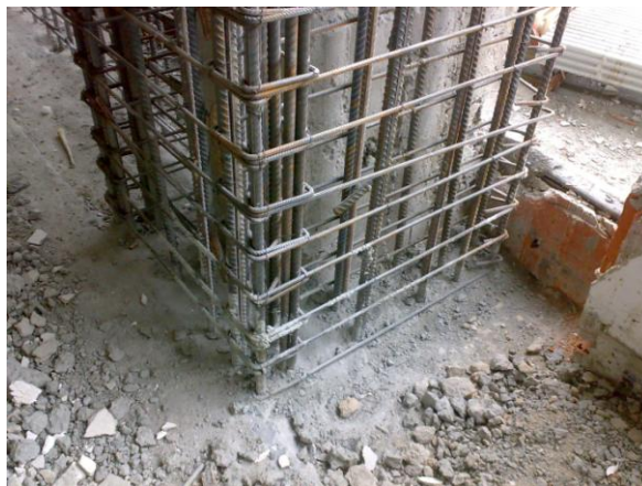
Figure 3.9. Reinforcement Details of the Column Jacket.
