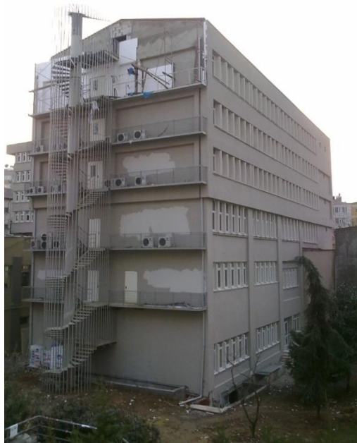
Figure 3.1. Overall View of the ET-B Building from the North-East Direction.
