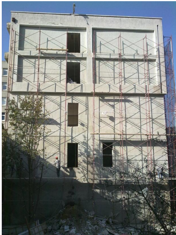
Figure 3.5. View of the Building after Strengthening, from East.
