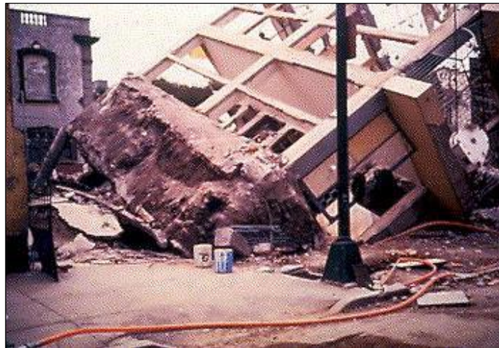
Figure 1.1. Building toppled due to lack of seismic bearing capacity during Mexico City Earthquake- Mexico (1985) (Merlos and Romo, 2006).
