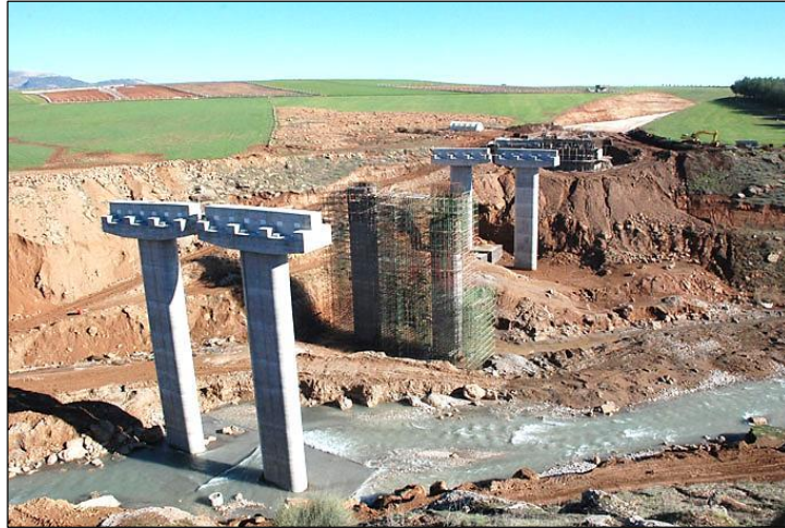
Figure 1.2. Bridge abutment constructed on top of slope (Ziyaret Bridge, Adiyaman, Turkey).
