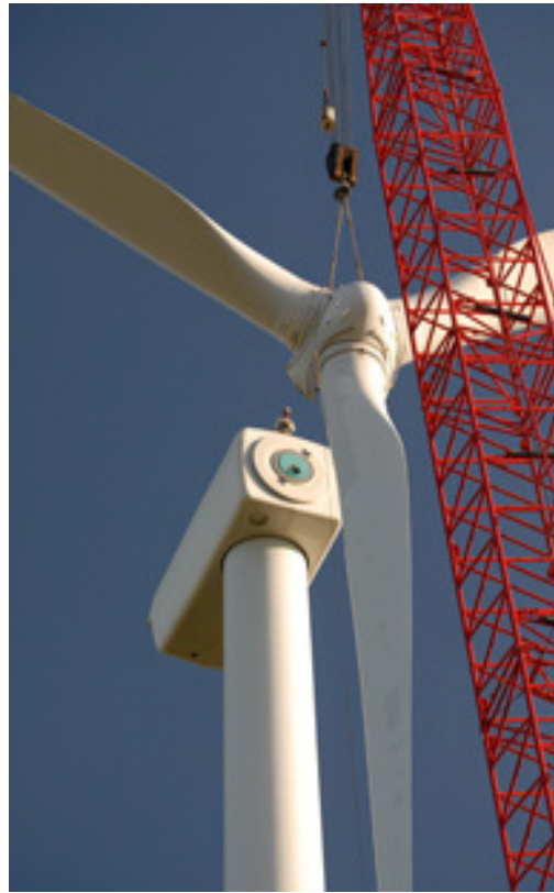
Figure 2.2. Rotor-Nacelle assembly
