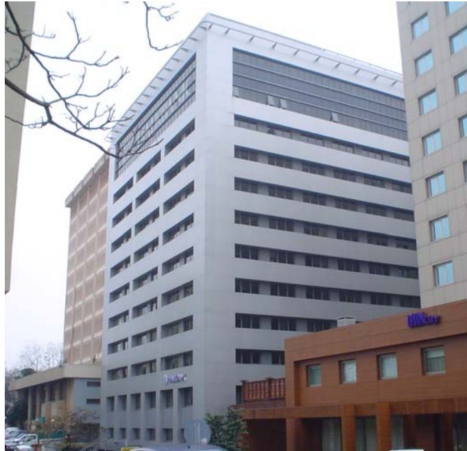
Figure 2.1. Photograph of the existing high-rise office building
