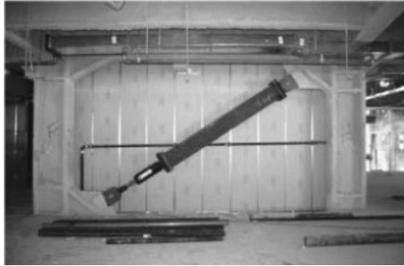
Figure 2.7. Installation of fluid viscous damper (Uriz and Whittaker, 2001)
