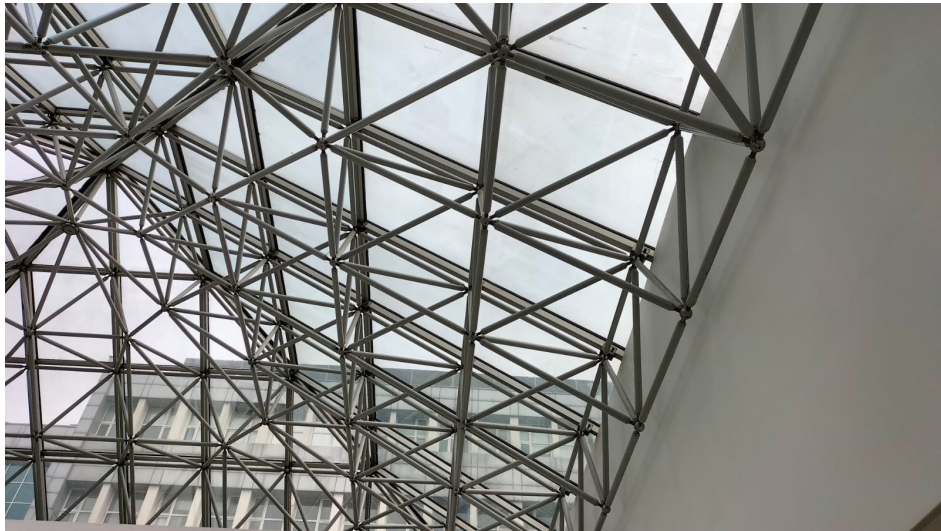
Figure 4.1. A generic truss structure.
