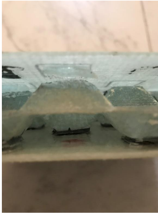
Figure 6.5. Split-off between the top face and the core section of the sandwich structure.
