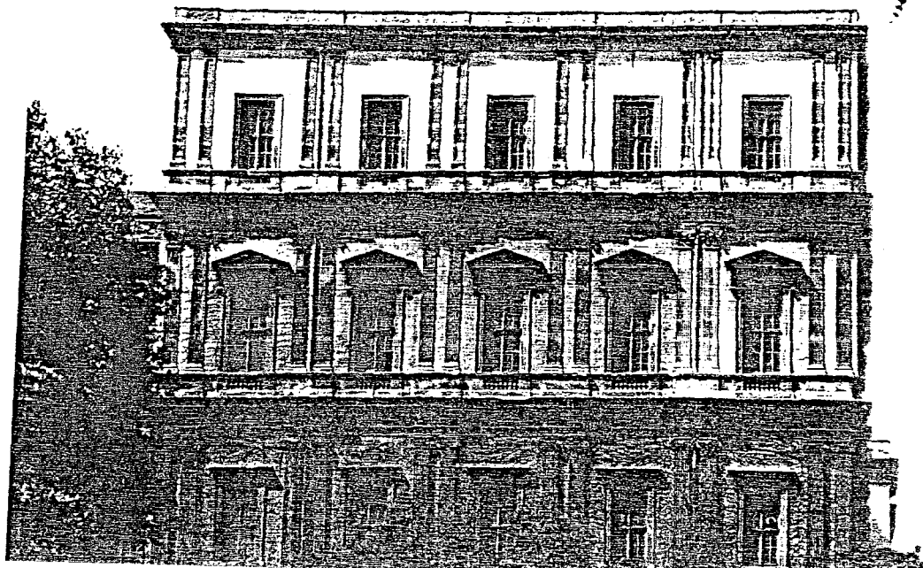
Fig. 8 View from South
