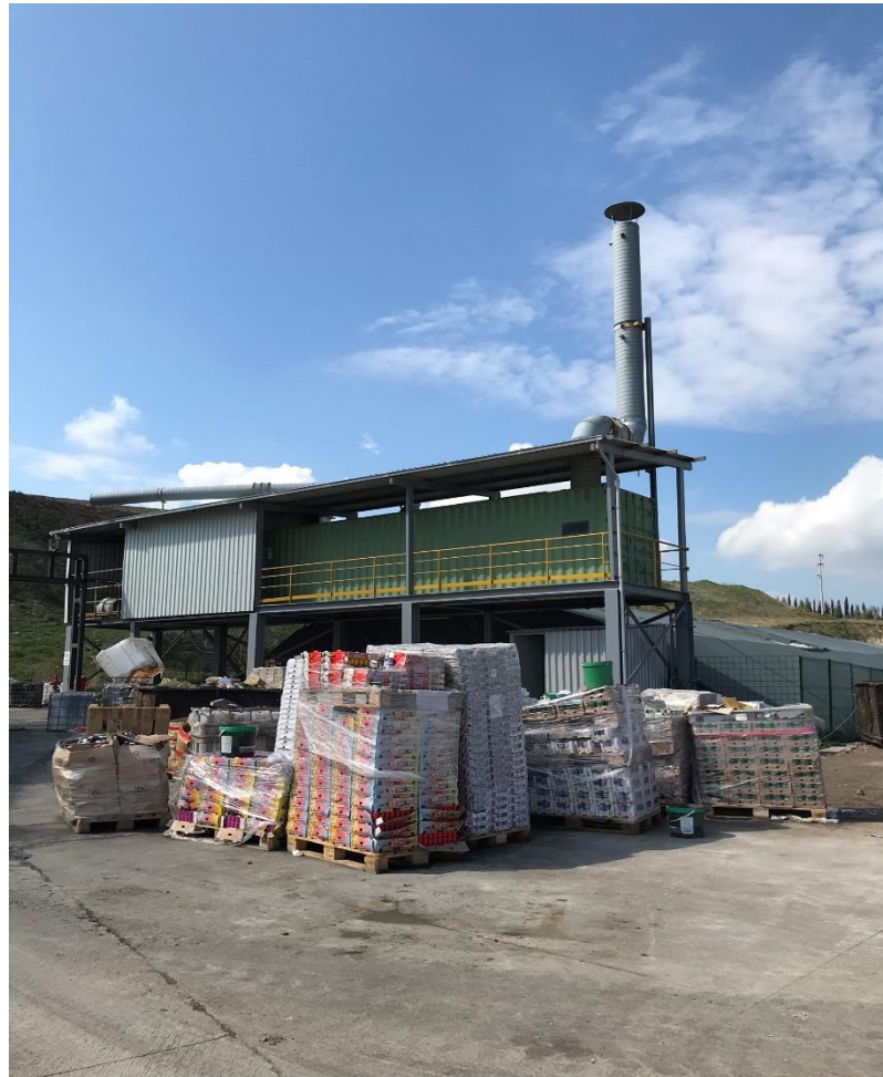
Figure B.4. Palletized wastes.
