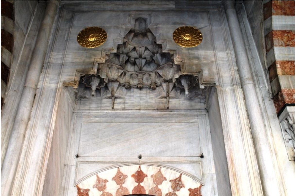
35. The muqarnas voussoir of the mausoleum of Murad III (Photography by the author)
