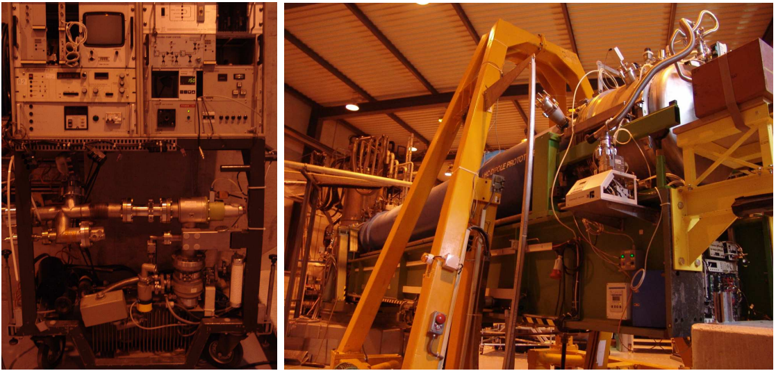
Figure B.2. Left: The Bonjon pump. Right: The differential pumping station
