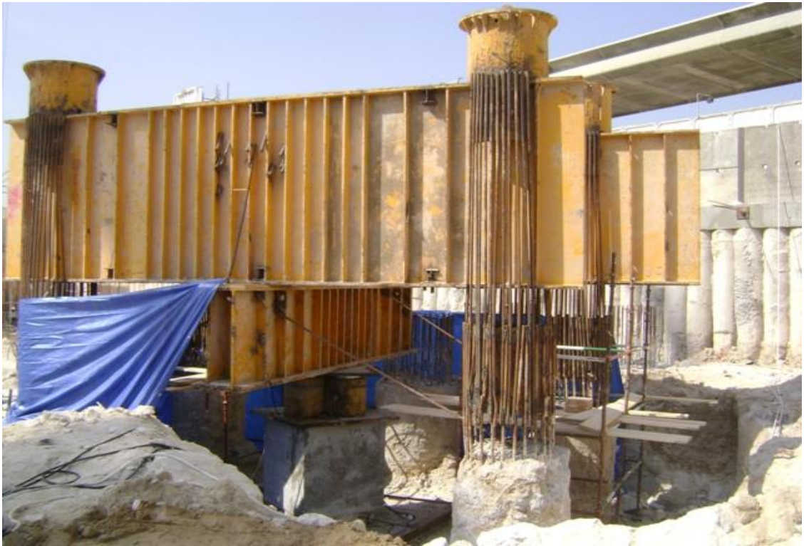
Figure 6.14. Test pile preparation
