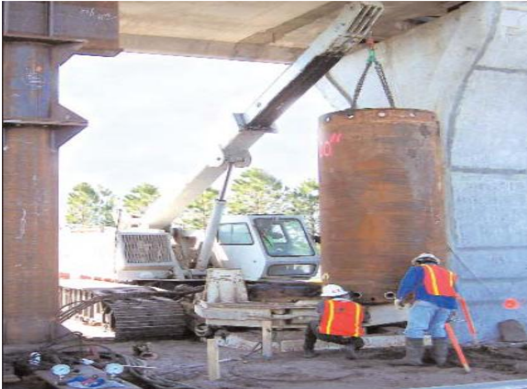
Figure 4.6. Casing oscillator used to advance casings down to the limestone (H. Beck Foundation Co., Inc.)
