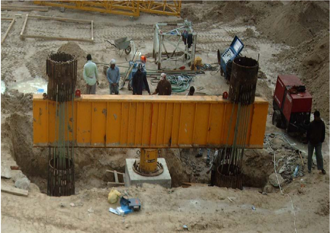
Figure 6.46. Static compression load test setup sample photo
