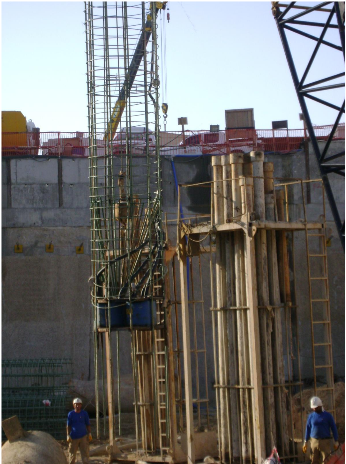
Figure 6.32. Installation of steel cage carrying the load cell
