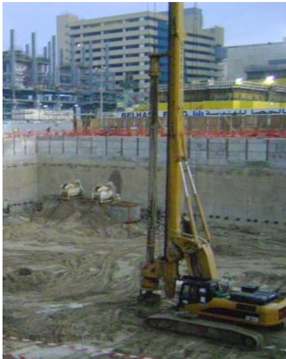
Figure 4.3. Piling rig machine (IMT AF220) Figure 4.4. Rig machine (Bauer BG28)
