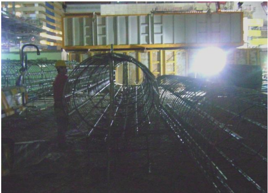
Figure 4.2. Steel cage preparation
