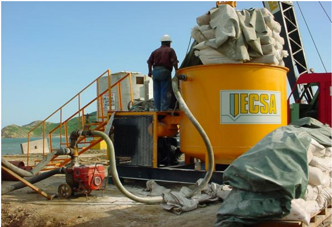
Figure 4.9. Bentonite slurry mixers (IECSA Co., http://www.iecsacv.com/graphics/eb/DSC00112.jpg )
