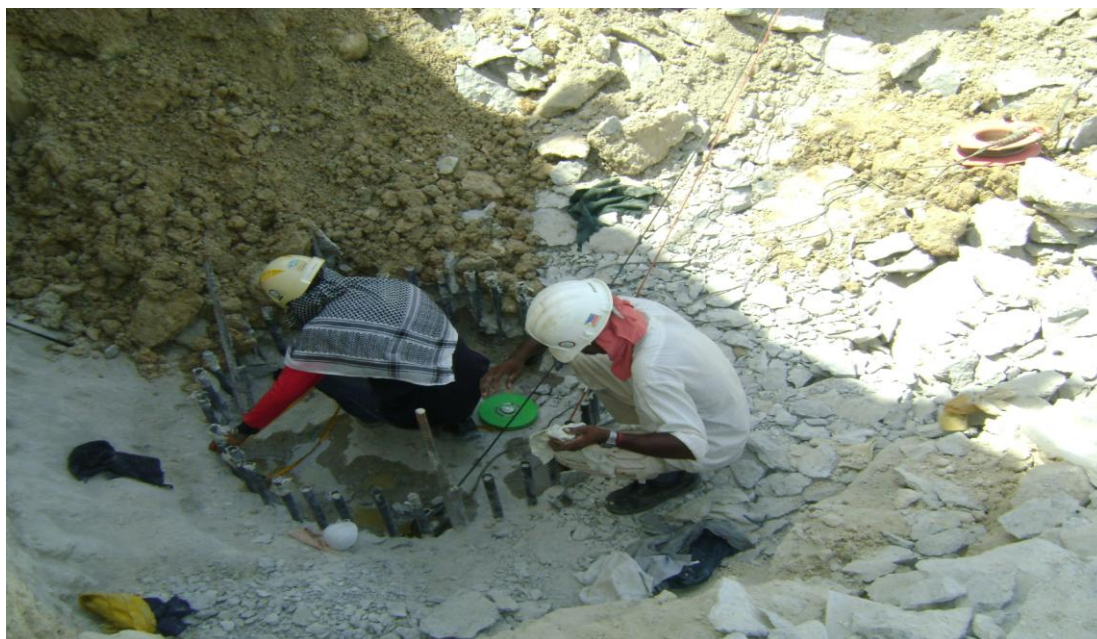
Figure 6.55. Installing transmitter cables down the access tubes
