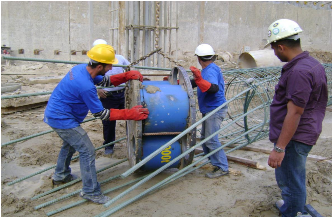
Figure 6.29. Installation of the load cell into steel cage
