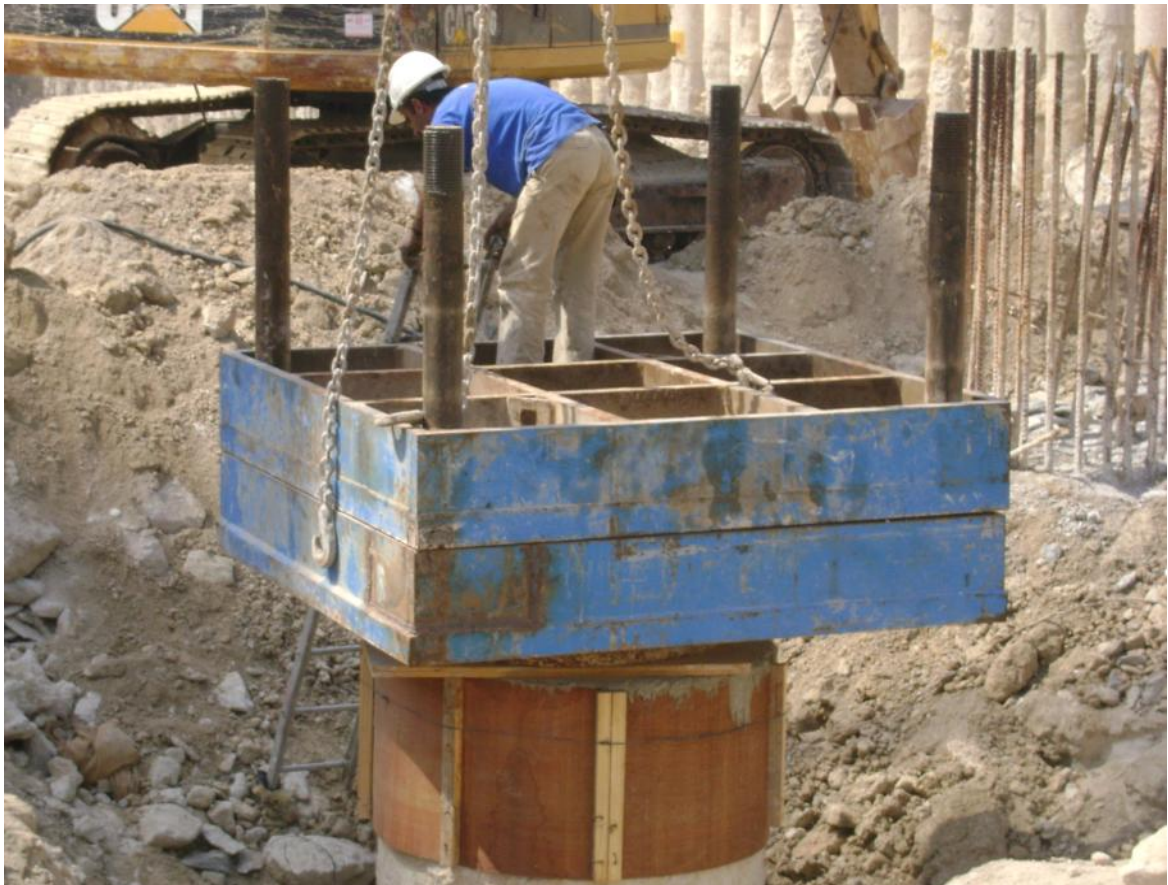
Figure 5.33. Installing drop weights
