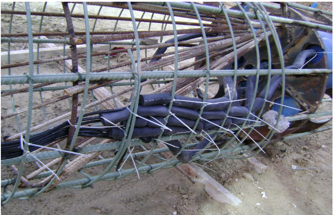
Figure 6.30. Positioning of the hydraulic load cell system
