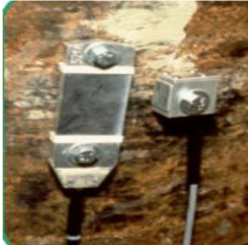
Figure 5.35. Strain transducer and accelerometer mounted on a pile ( http://www.whitakerlab.net )
