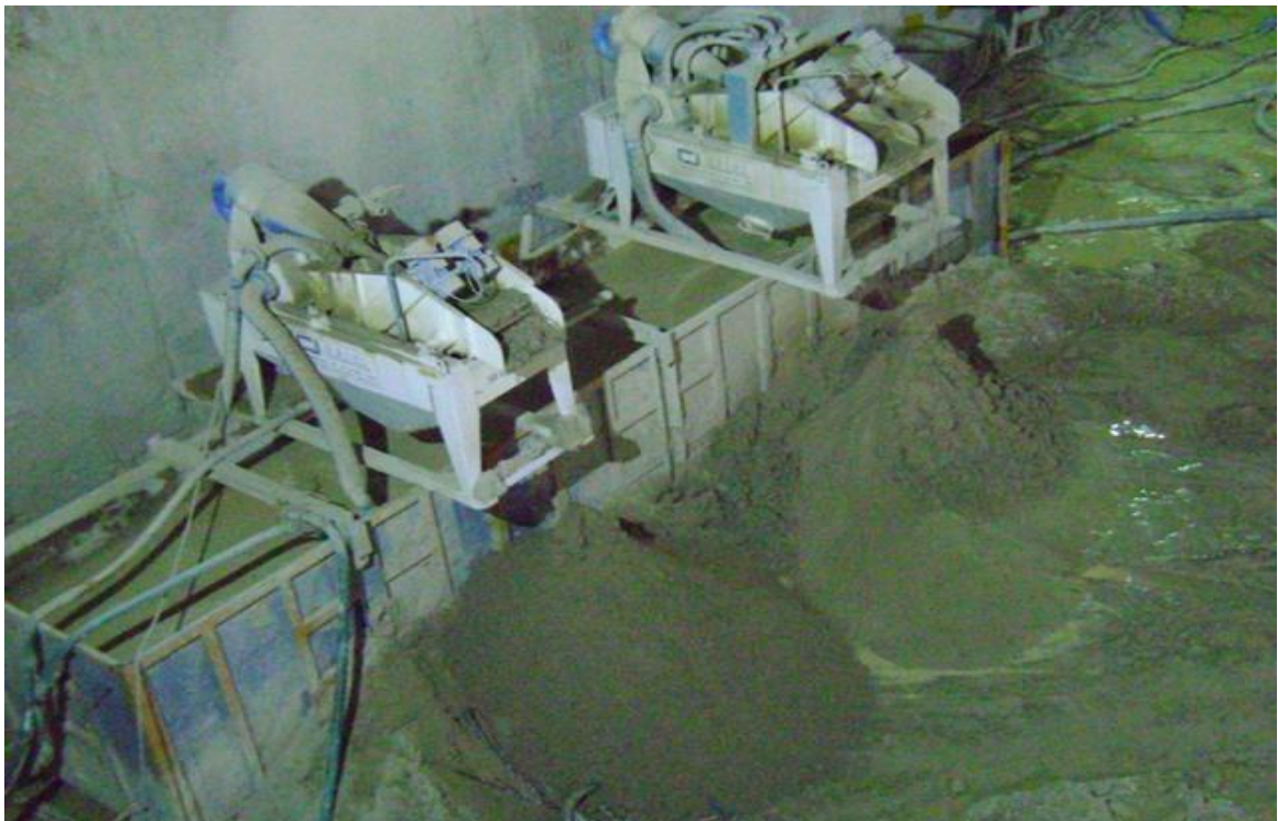
Figure 4.12. Stabilizing fluid, bentonite preparation and storage
