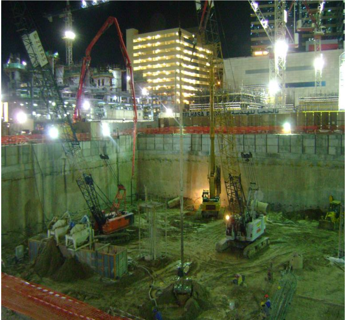
Figure 4.15. Pile casting
