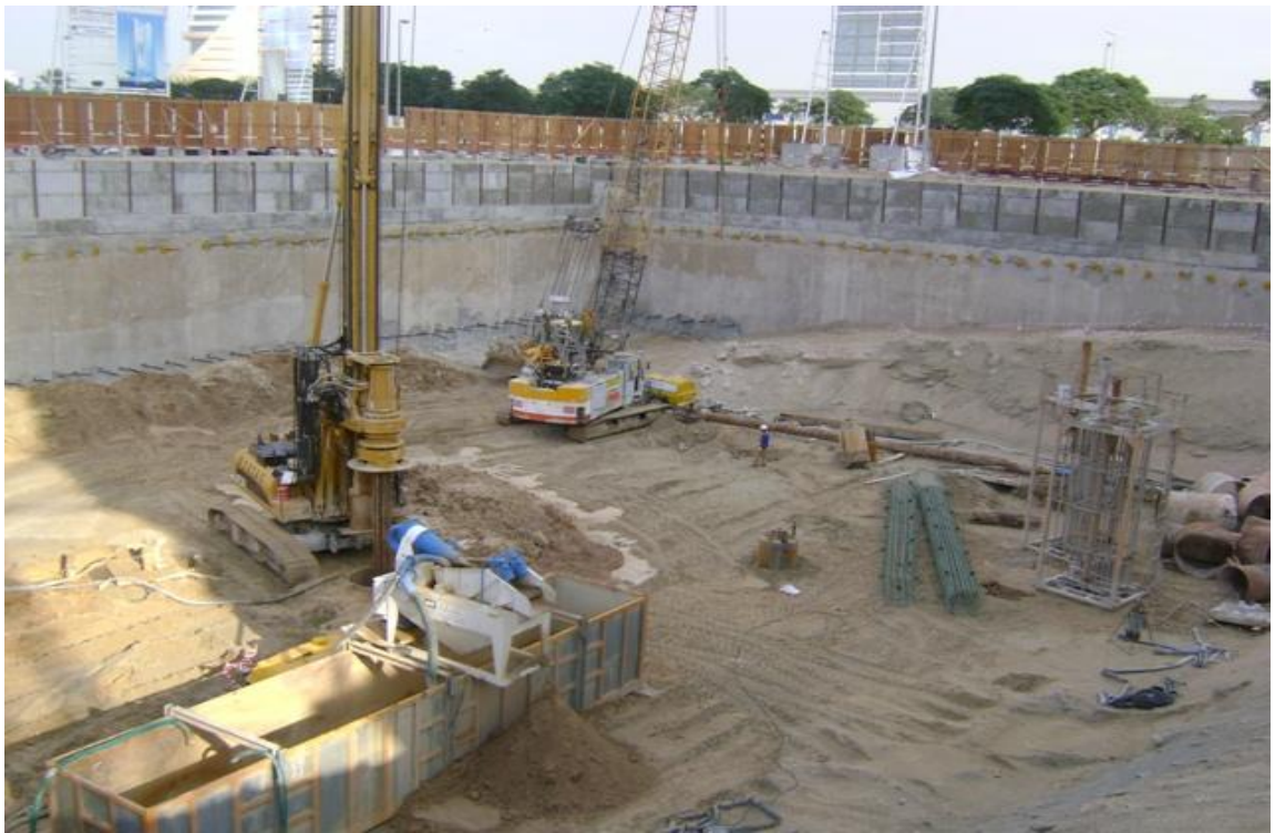
Figure 6.3. Construction in day shift
