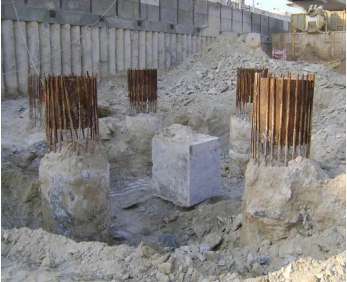
Figure 5.3. Pile head preparation for the static loading test
