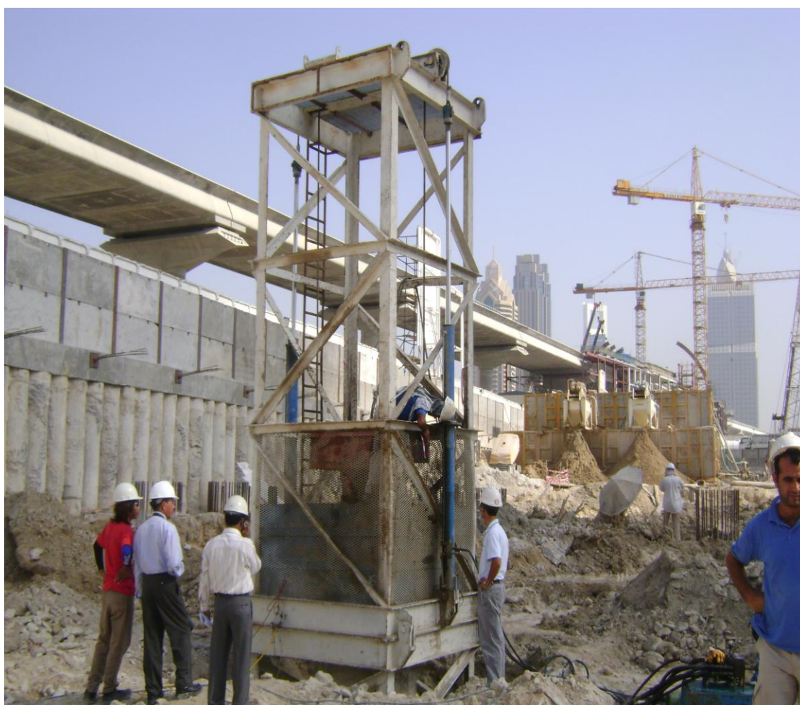
Figure 6.51. Dynamic test preparation
