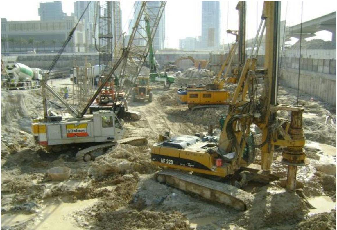
Figure 4.10. Guide casing installed bored pile excavation
