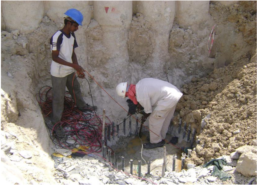
Figure 5.39. Probe installation for cross-hole test
