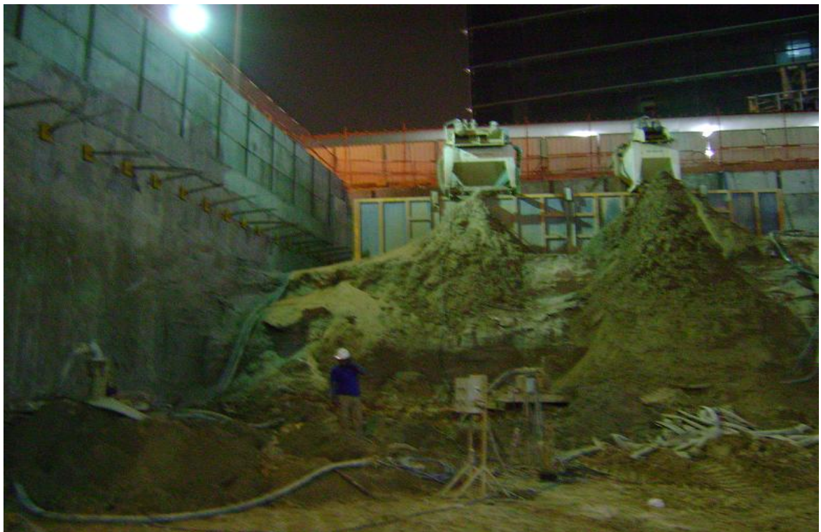
Figure 4.14. Flushing of borehole by desanders
