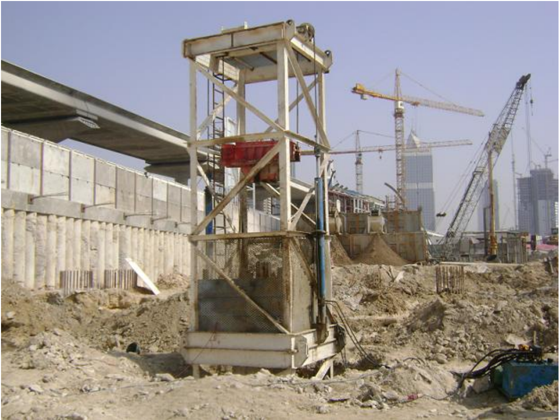
Figure 5.28. Dynamic testing overview
