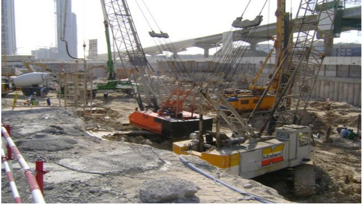
Figure 6.23. Construction in day shift
