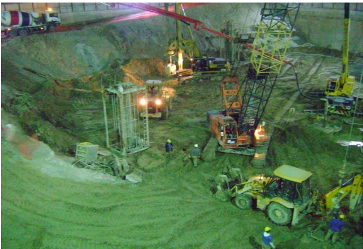
Figure 6.4. Construction in night shift
