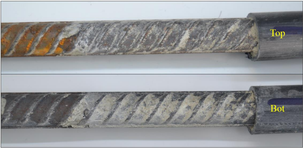
Figure 4.36. Mortar adhered on bars in a column specimen of RCAC.
