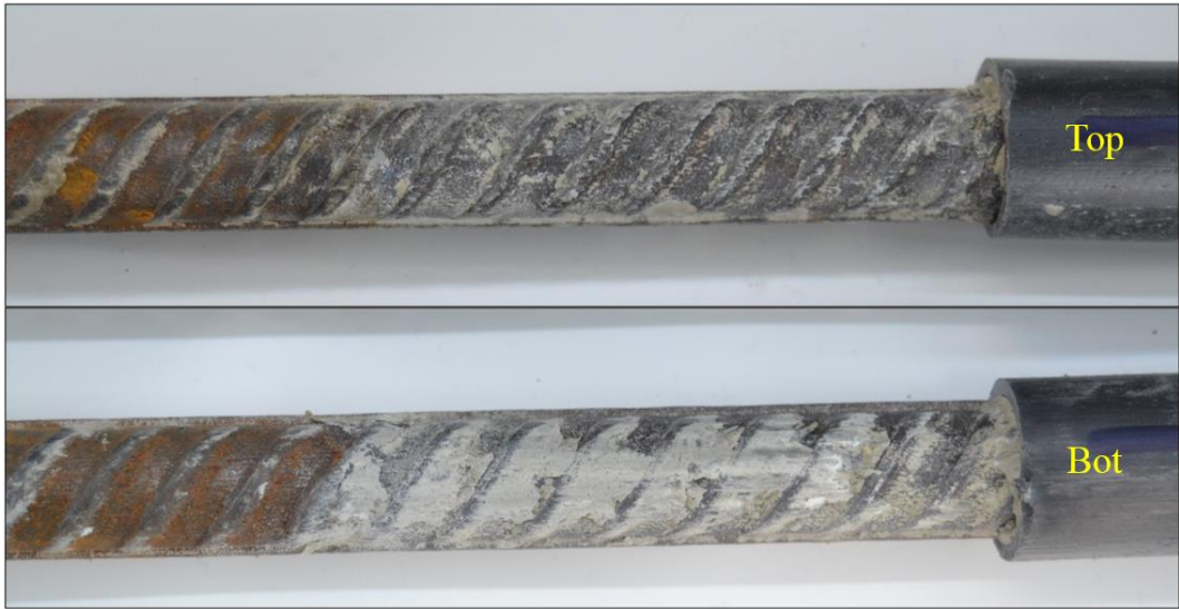
Figure 4.34. Mortar adhered on bars in a column specimen of FAAC.
