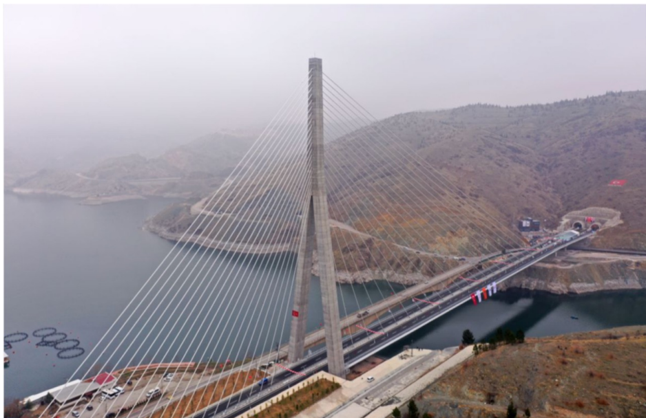
Figure 3.1. General view of New Kömürhan Bridge.
