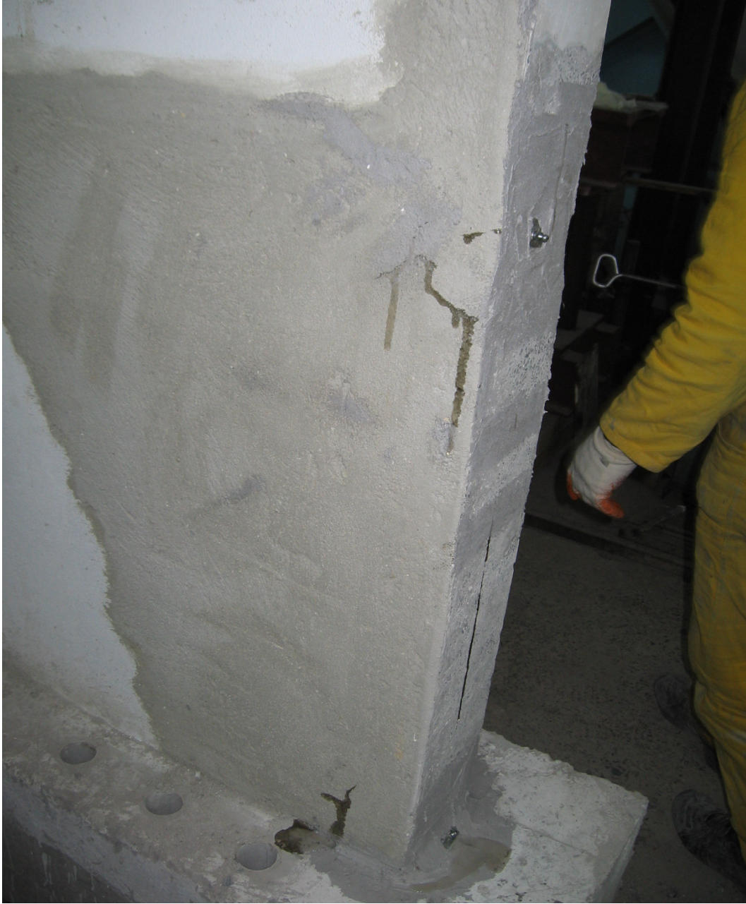
Figure 3.14. The flow-out of epoxy resin after injection for Specimen O2
