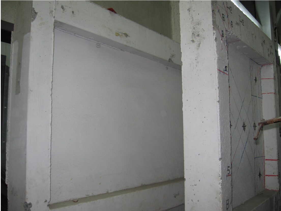
Figure 3.5. Second floor of test specimens
