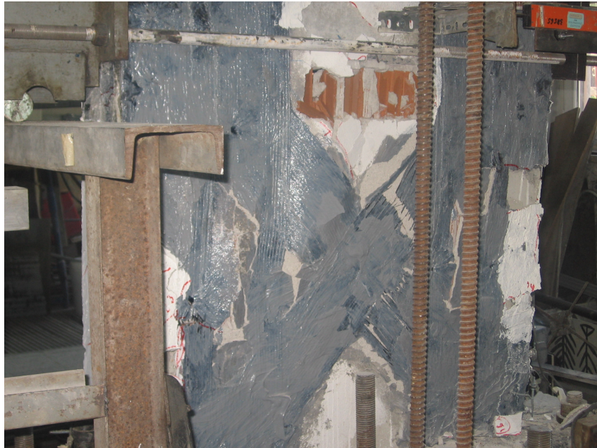
Figure 4.3. Rupture of diagonal and vertical FRP for specimen O1
