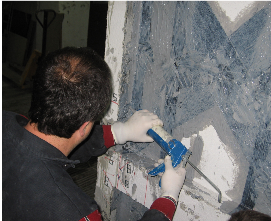
Figure 3.22. Filling the anchorage holes with epoxy resin
