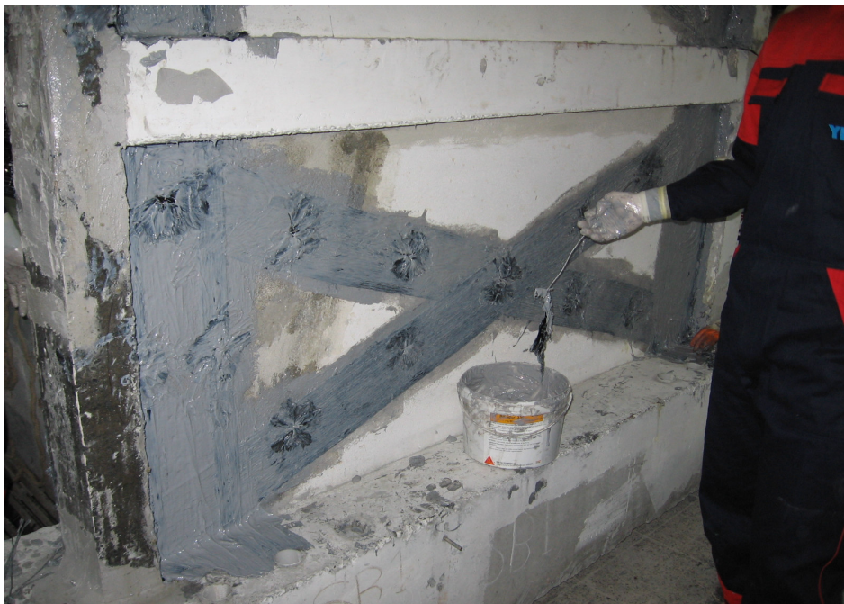
Figure 3.19. Anchorage application for specimen O2
