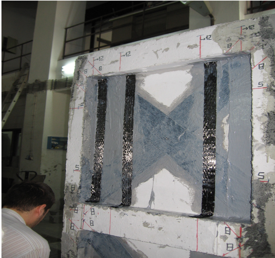
Figure 3.18. Vertical and cross FRP application specimen O1
