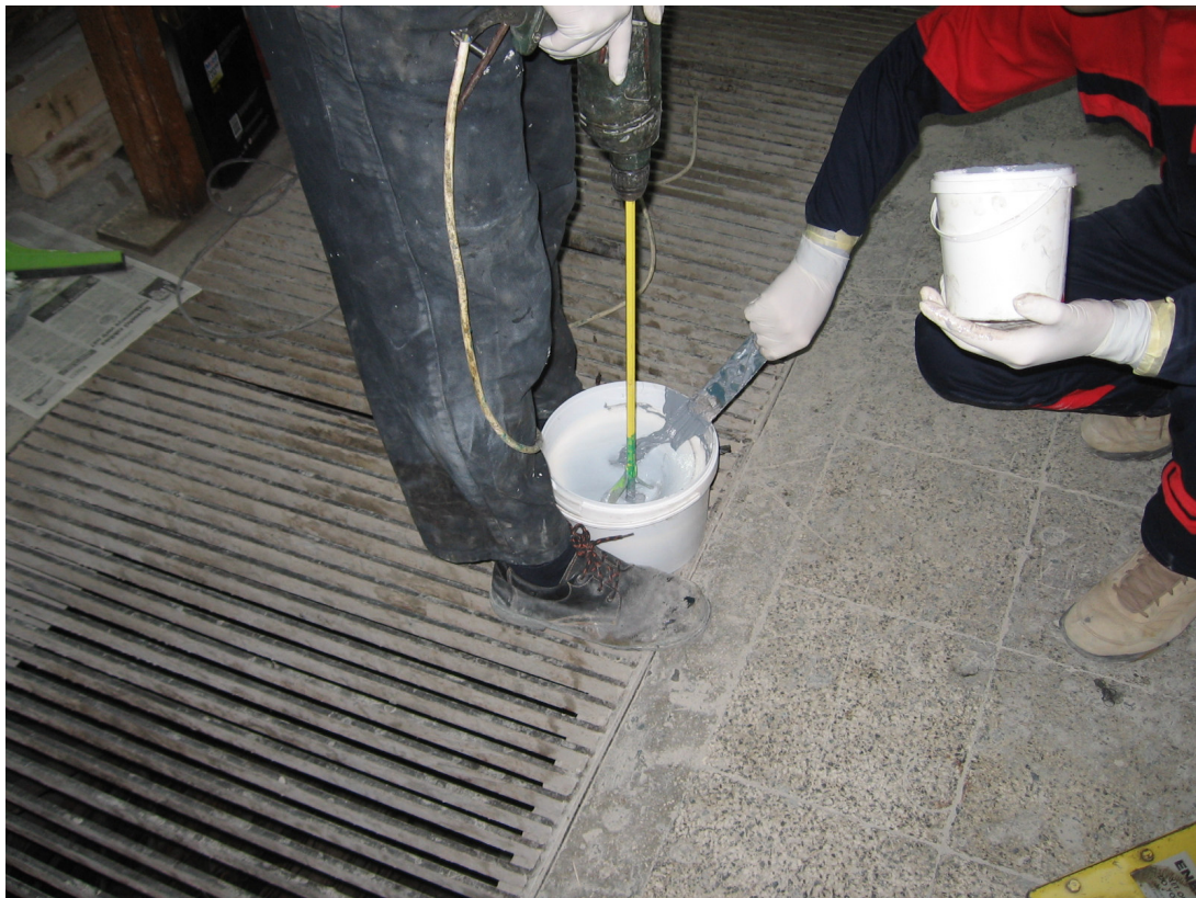
Figure 3.17. The preparation of the two-component epoxy impregnation resin
