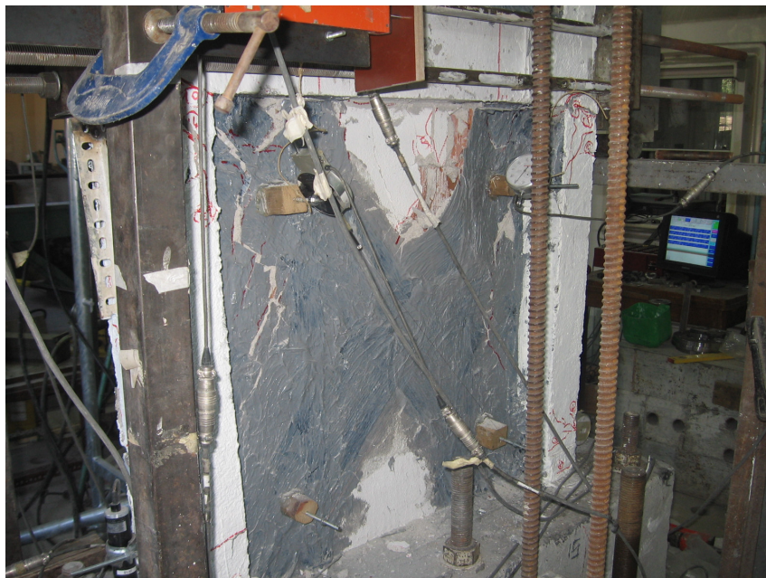
Figure 4.4. Debonding of diagonal FRP for specimen O1
