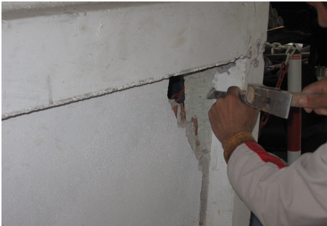
Figure 3.6. Roughing of concrete surface
