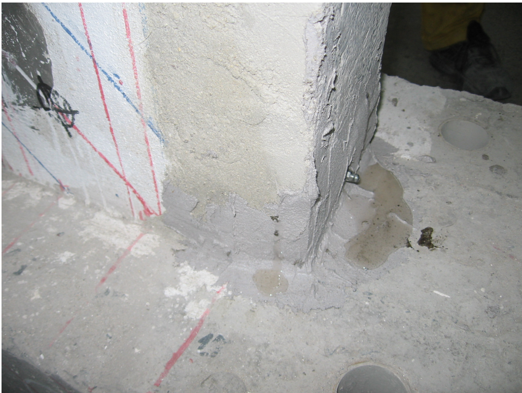
Figure 3.16. The flow-out of epoxy resin after injection for specimen O1
