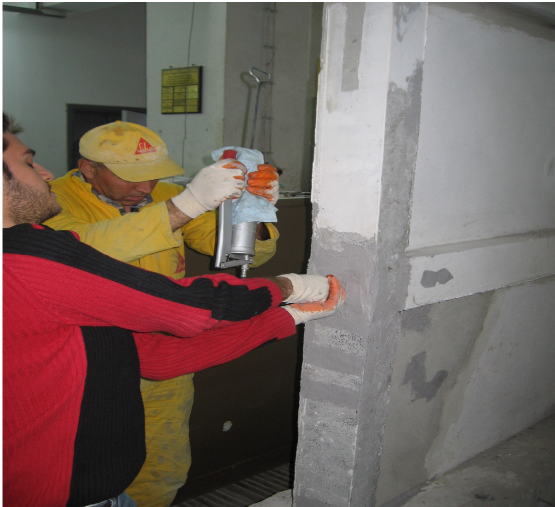
Figure 3.13. Pumping the epoxy resin for specimen O2
