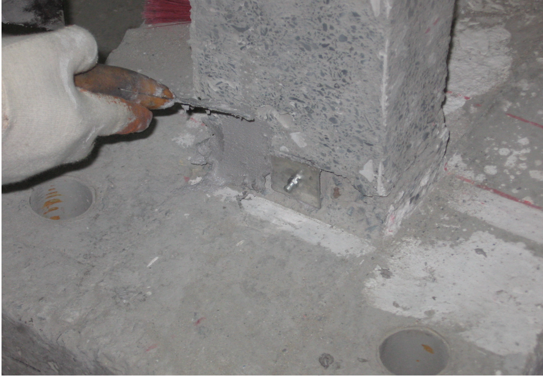
Figure 3.11. Placement of injection dowel
