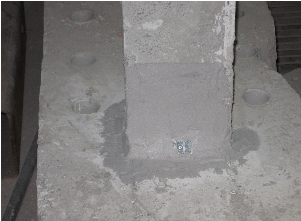
Figure 3.12. Finished application of Sikadur 31 and injection dowel
