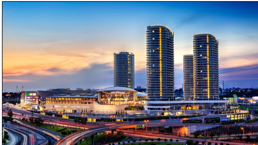
Figure 2.1. An illustration of multiple buildings sharing the same geometrical and structural properties (Mall of Istanbul project, residence blocks)
