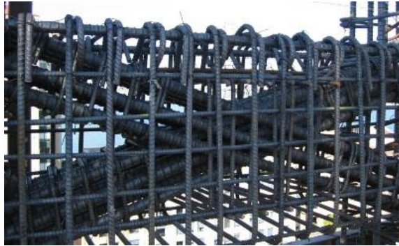
Figure 2.5. Diagonal reinforcement configuration in a coupling beam
