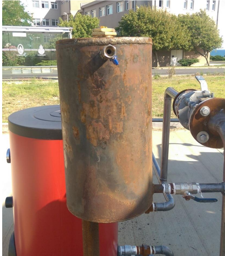
Figure 3.7. Expansion tank.
