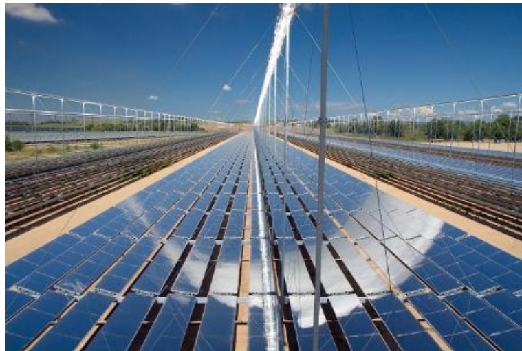
Figure 1.3. Linear fresnel [13].
