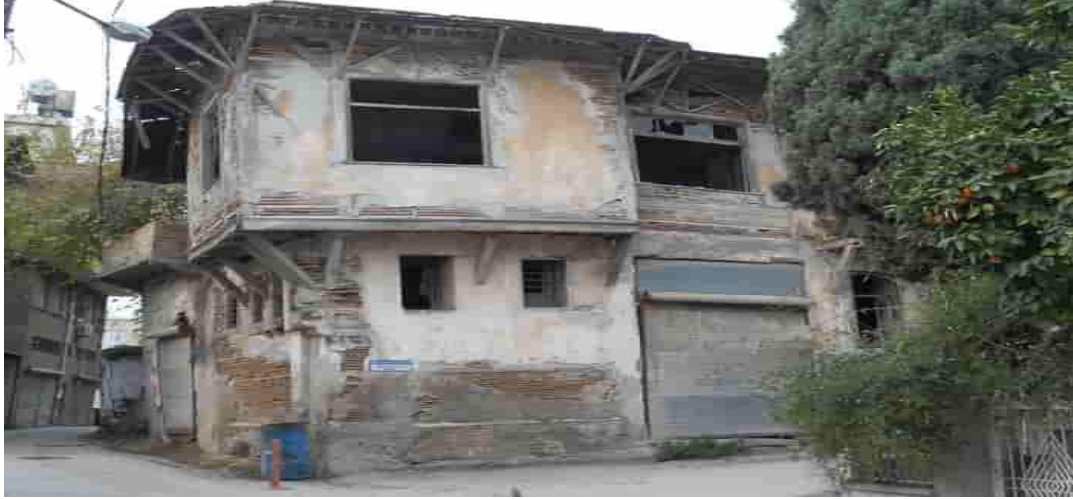
Figure 3. A Tepebağ House
