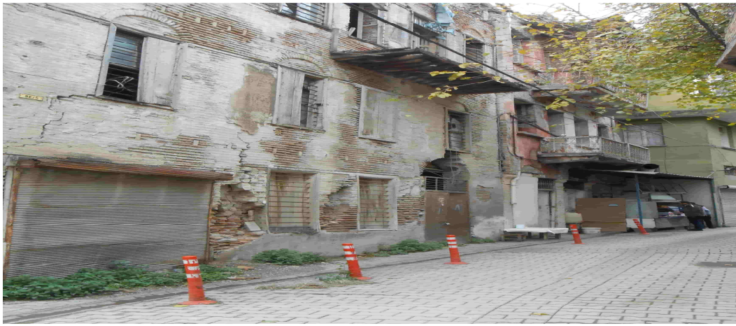
Figure 4. A Tepebağ House
