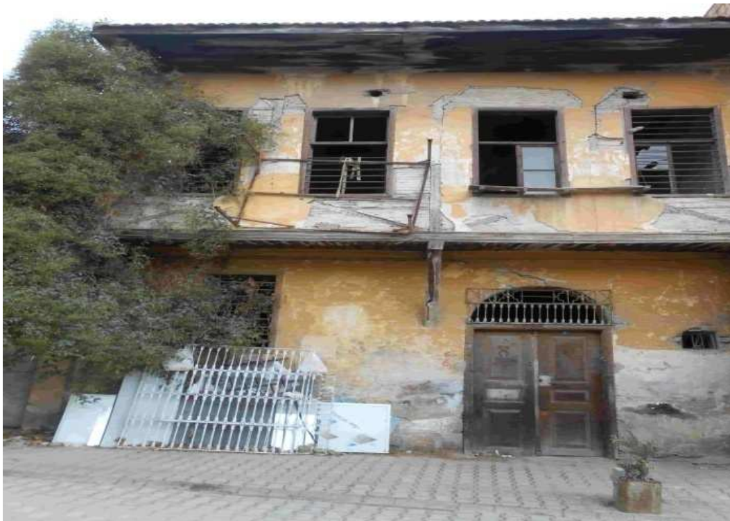
Figure 2. A Tepebağ House
