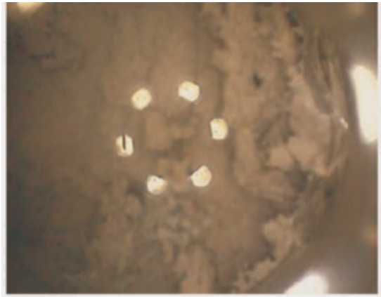
(i) Overcut gap photo near to bentonite injection port.
