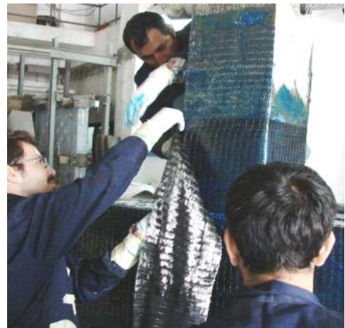
Figure 3.14. Application of column wraps
