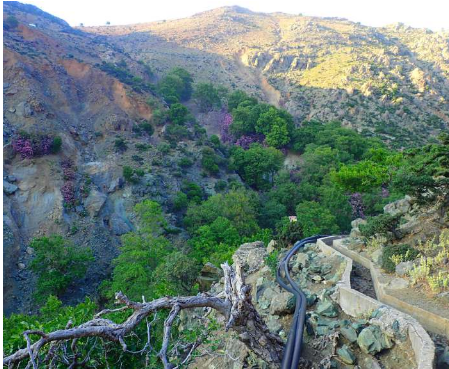
Figure 4.15. Individually Plotted PVC Pipes at an Abandoned Aqueduct, Xiropotamos Basin.
