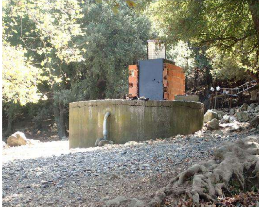
Figure 4.10. Cistern Installed at Spring Outflow. Source: Skoulikidis et al. 2019
