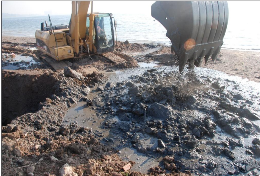
Figure 3.2. Test pit opened 10 m landward from the shoreline: at 5 m depth still fill material was observed.
