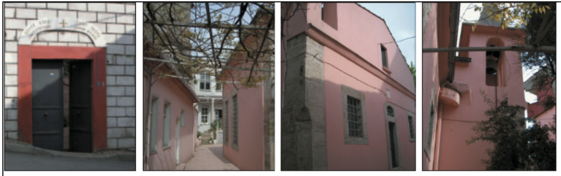
Figure 19. Surp Yeghia Church’s entrance from the street, courtyard, eastern façade and bell tower (Hañçer, “Eyüp Ermeni kiliseleri.”)
