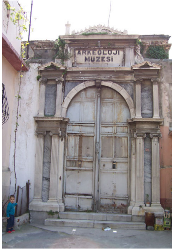
Image 3. The main entrance gate of the courtyard, which still has the name of the museum on top.
