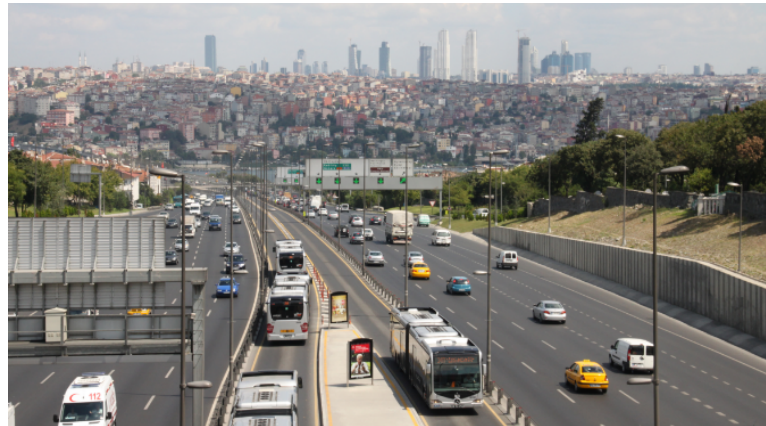
Figure 4.11. D100 Highway after the implementation of the BRT line [100].
