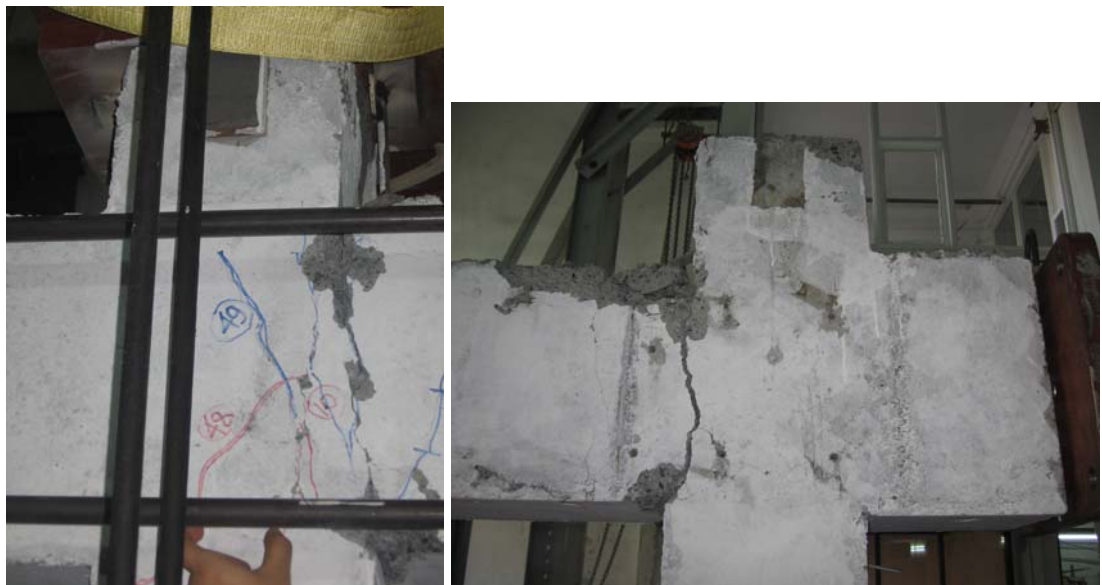
Figure 3.4. Joint Shear Cracks and Beam Crushing
