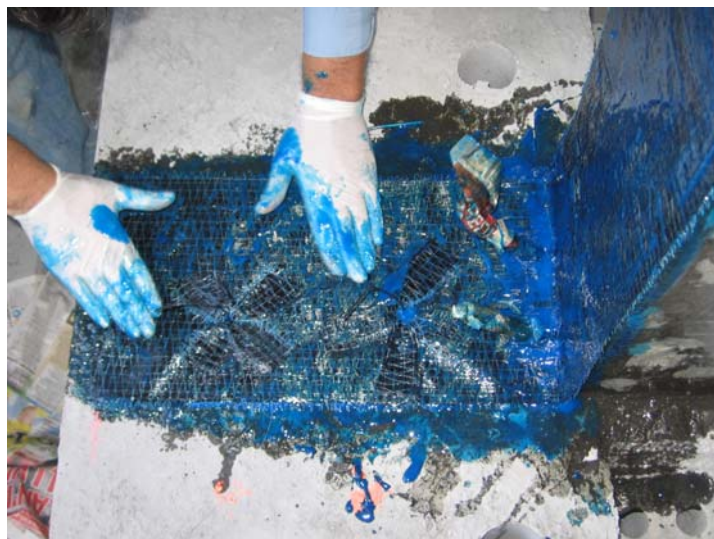
Figure 2.22. CFRP Anchorages
