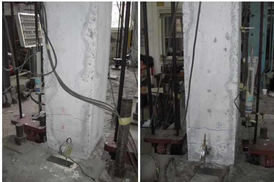
Figure 3.3. Column Flexural Cracks (exterior and interior)
