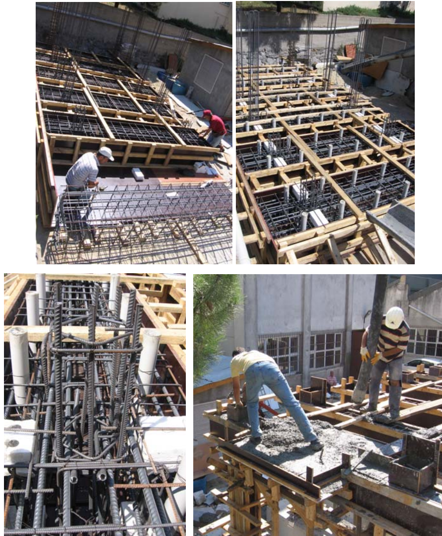
Figure 2.13. Production of Test Specimens
