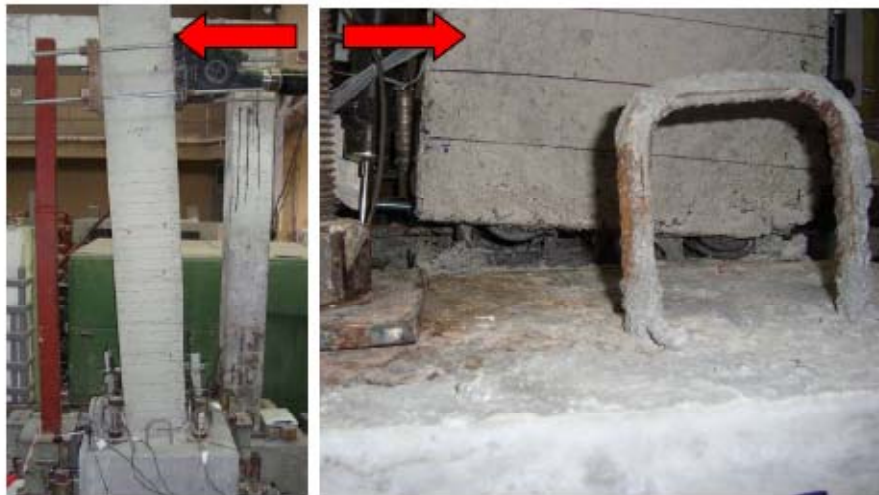
Figure 8.60. Damage at the Base of Specimen LS-44φ-N1 (Yilmaz, 2009).
