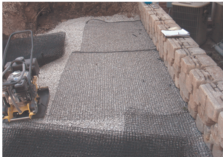
Figure 3.4. Geogrid as an extensible reinforcement.
