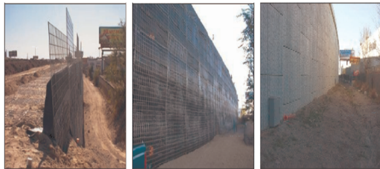
Figure 4.28. Photographs of the MSE wall constructed at 3600 South and I-15 (Budge et al. , 2006).
