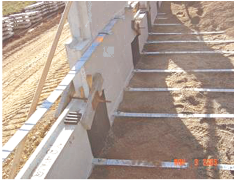
Figure 3.3. Metal strip as an inextensible reinforcement.
