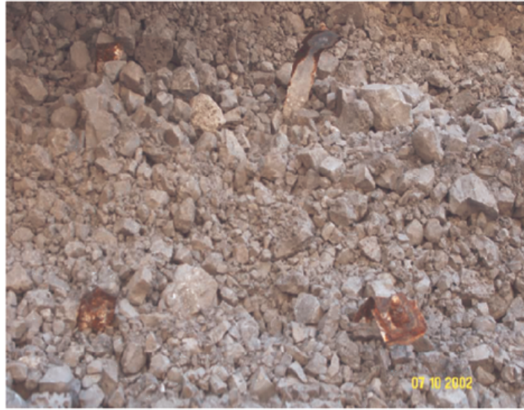
Figure 4.32. Corroded metallic soil reinforcements (Armour, 2004).
