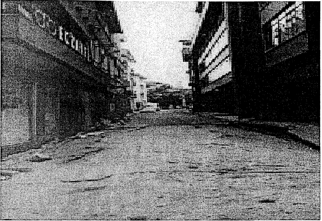
Figure 2-7 Liquefaction-Induced Settlement of Adjacent Buildings and the Uplift of the Sewage System Pipe (NZSEE, 1999)
