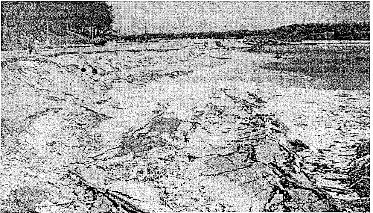
Figure 2-3 A Small Flow Slide along the Shore of Lake Merced in San Francisco in 1957
