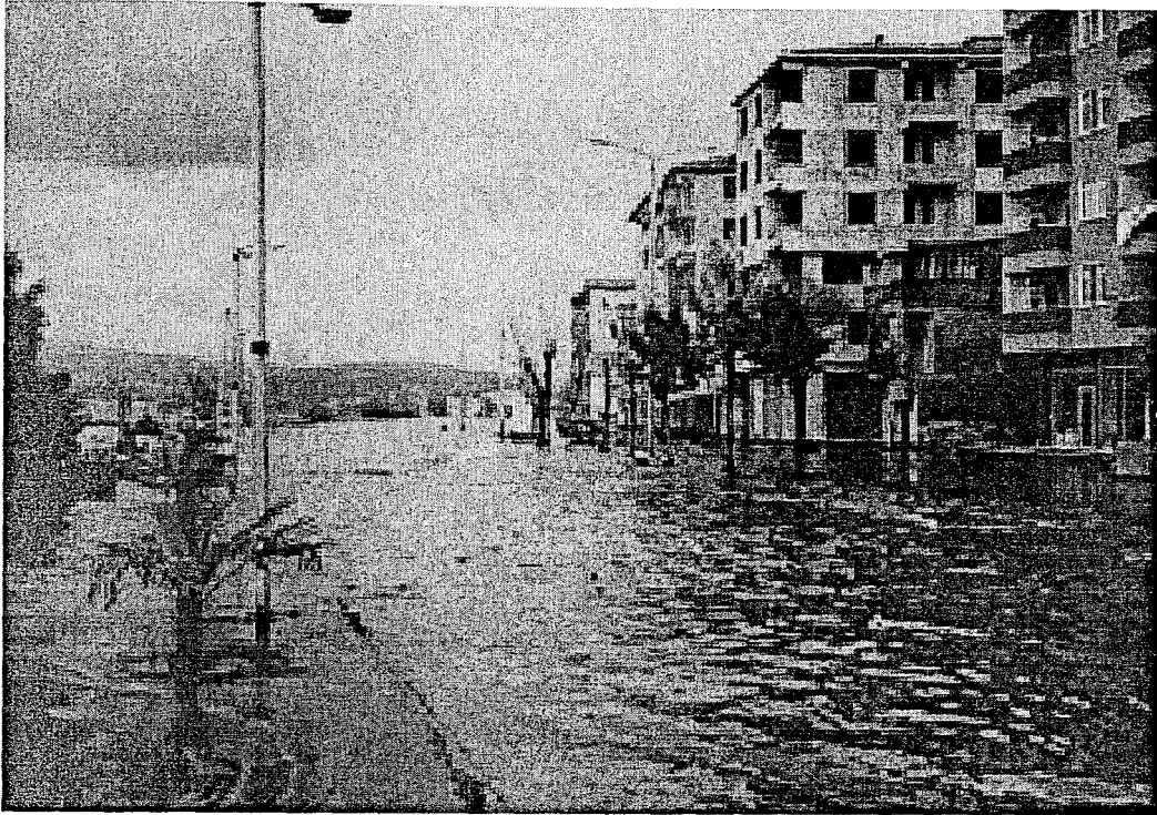
Figure 2-15 Lateral Spreading and Settlement Example from Gölçük (NRC,1985)
