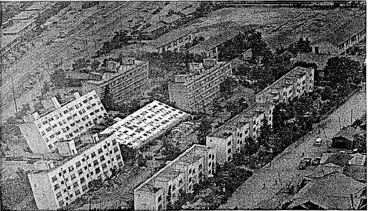
Figure 2-6 Liquefaction Failures in 1964 Niigata Earthquake (Steinbrugge Collection)
