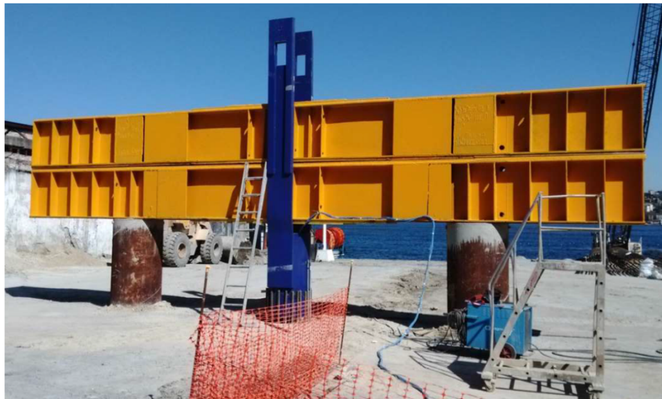
Figure 4.5. An example of pull-out test setup.
