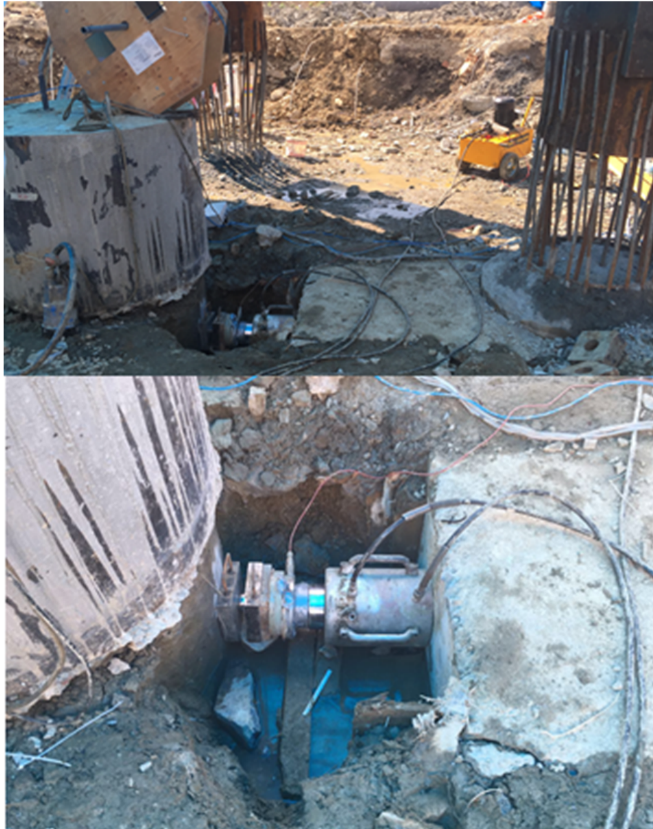
Figure 4.6. An example of lateral load test setup.
