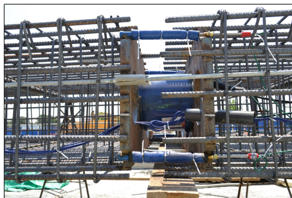
Figure 5.6. Osterberg load cells together with upper and lower plates.
