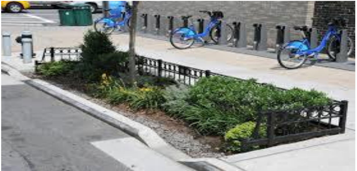
Figure 5.37. A bioswale in Binghamton, New York (Binghamton-ny.gov).
