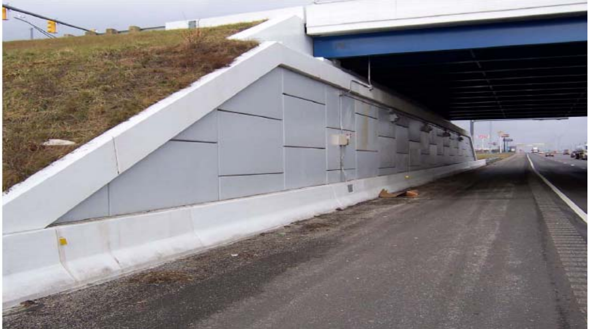
Figure 4.10. VSL wall application at USA (Tensar, 2006)
