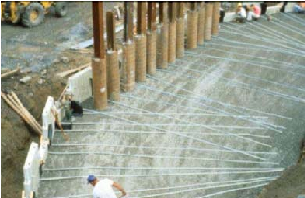
Figure 3.5. Construction with metallic strips (MSE Handbook, 2006)
