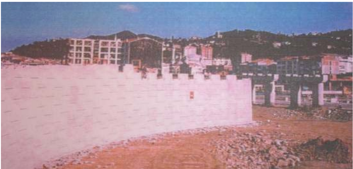
Figure 4.1. Reinforced earth retaining wall construction at Umraniye Istanbul (Demirkan, 2002)
