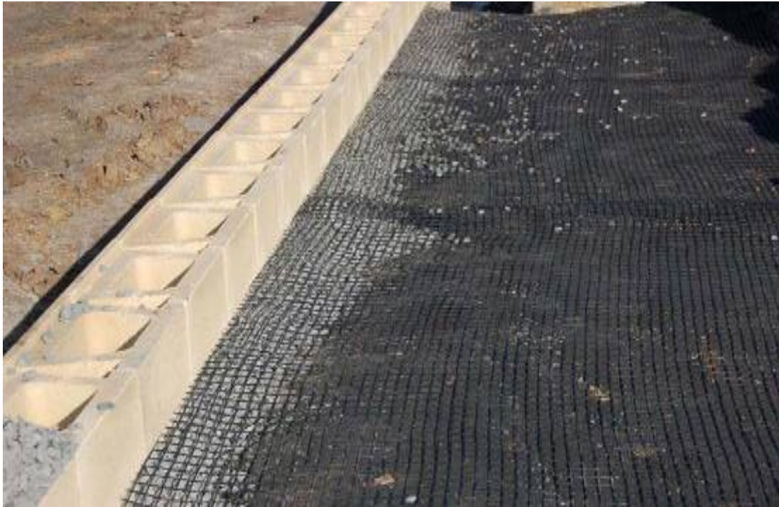
Figure 3.8. Geogrid reinforcement application (Koerner, 1998)
