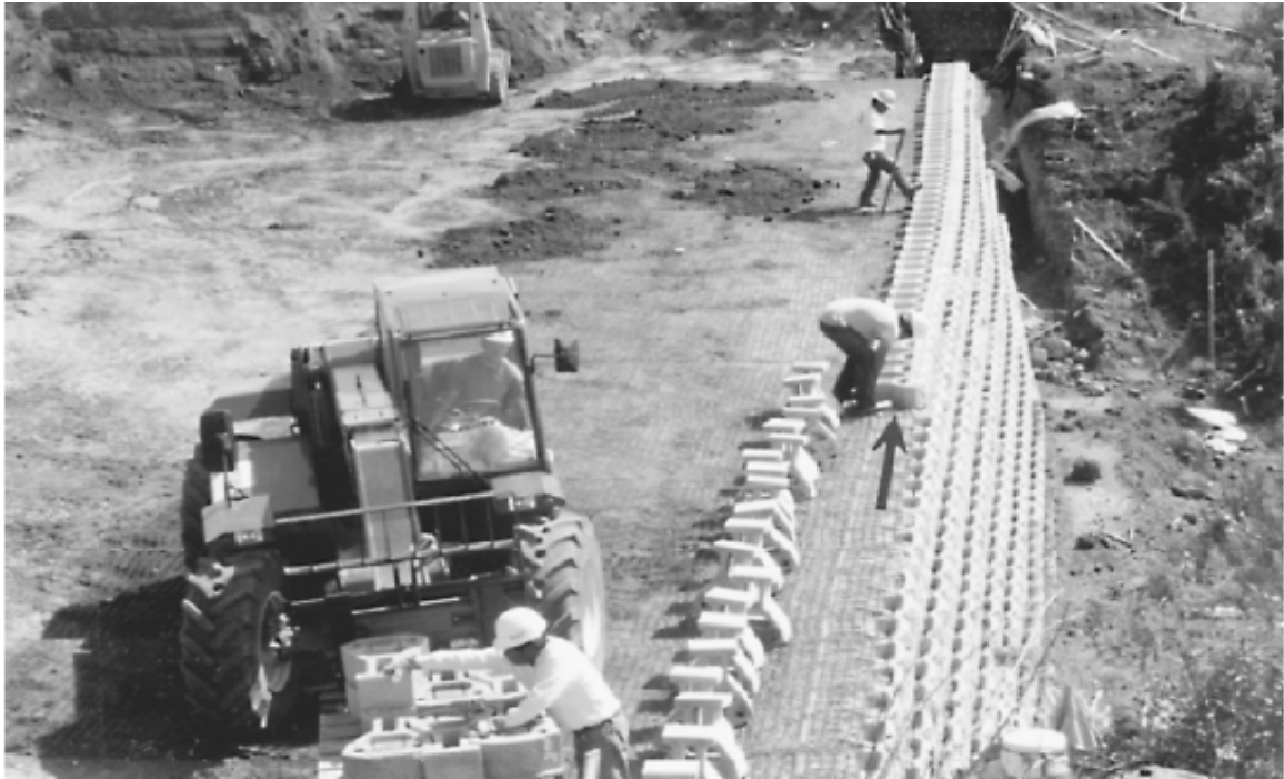
Figure 4.9. Installation of a mechanically stabilized earth retaining wall (Tensar., 2006)
