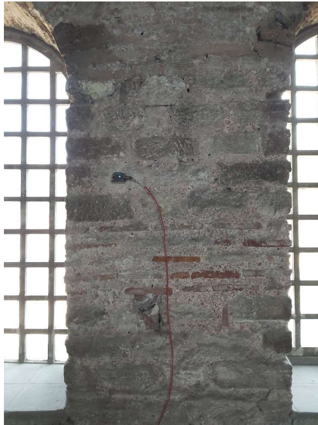
Figure 5.5. Accelerometer on the Wall
