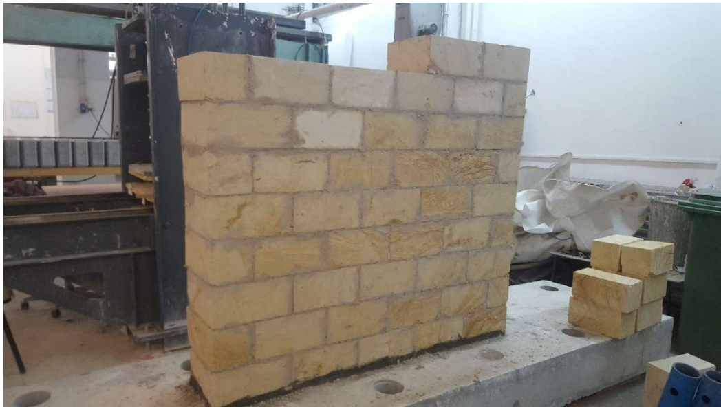
Figure 4.1. The Wall Under Construction
